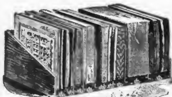
Shelf removed from Catalogue Cabinet, showing method of indexing.
