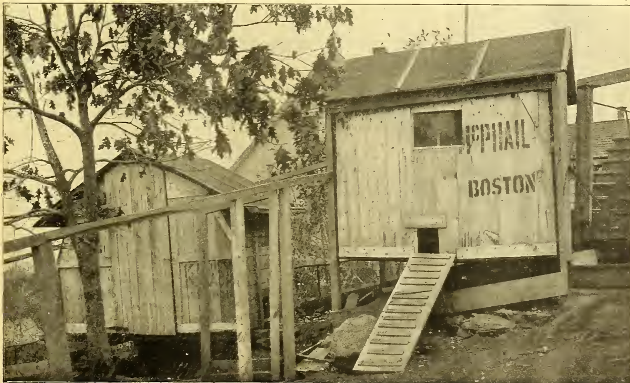
Poultry Houses made of two piano boxes. One house shows the end view; the other, the side view. These boxes cost but forty or fifty cents apiece. The roof is covered with tarred paper and the house complete is snug and secure.
