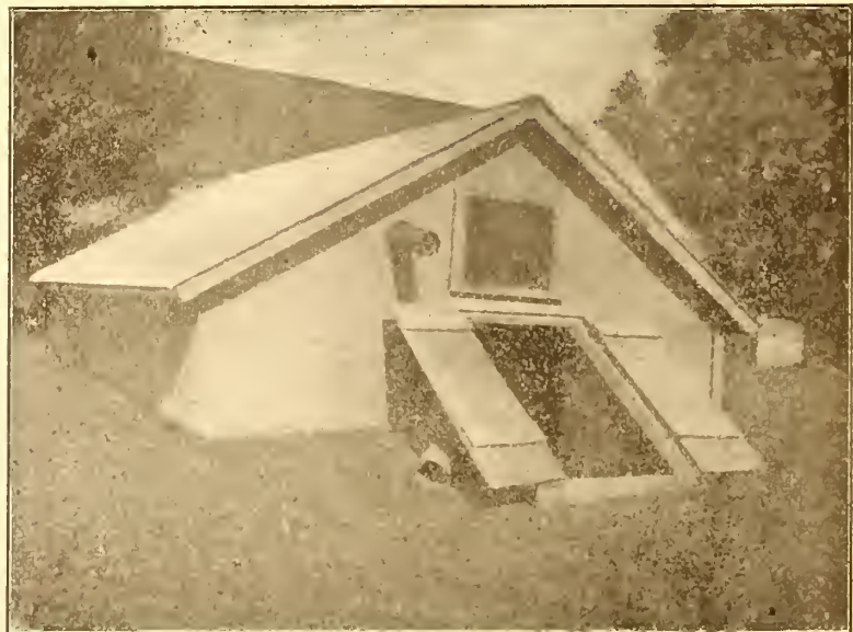
The incubator cellar built to accommodate six incubators—Imperial Poultry Farm, Valley Junction, Iowa.
