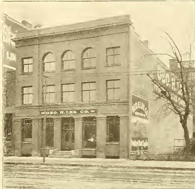
New factory built and owned by the Geo. H. Lee Co., Omaha, Nebr. Size, 44x130 feet, full three stories and basement. Walls are heavily built so more stories can be added when needed.
