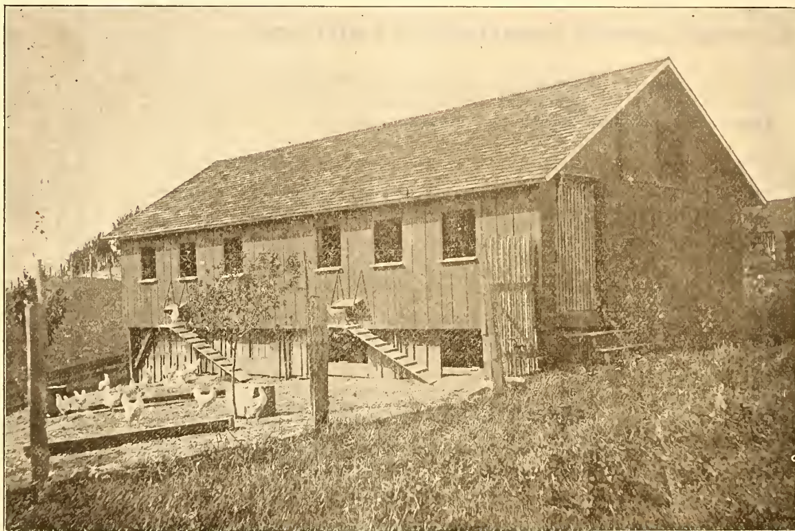
A house for yarded layers at the Fairview Farm, Groton, N. Y., Single Comb White Leghorn specialists. The basement is light and well ventilated, providing a resting and wallowing place during hot or stormy days of summer, and a scratching room during winter. The main floor is fitted with nests and roosts; the loft has twelve inches of straw on the floor which serves to absorb moisture during cold days. On mild days the gable ends of loft are opened to dry out the straw.
