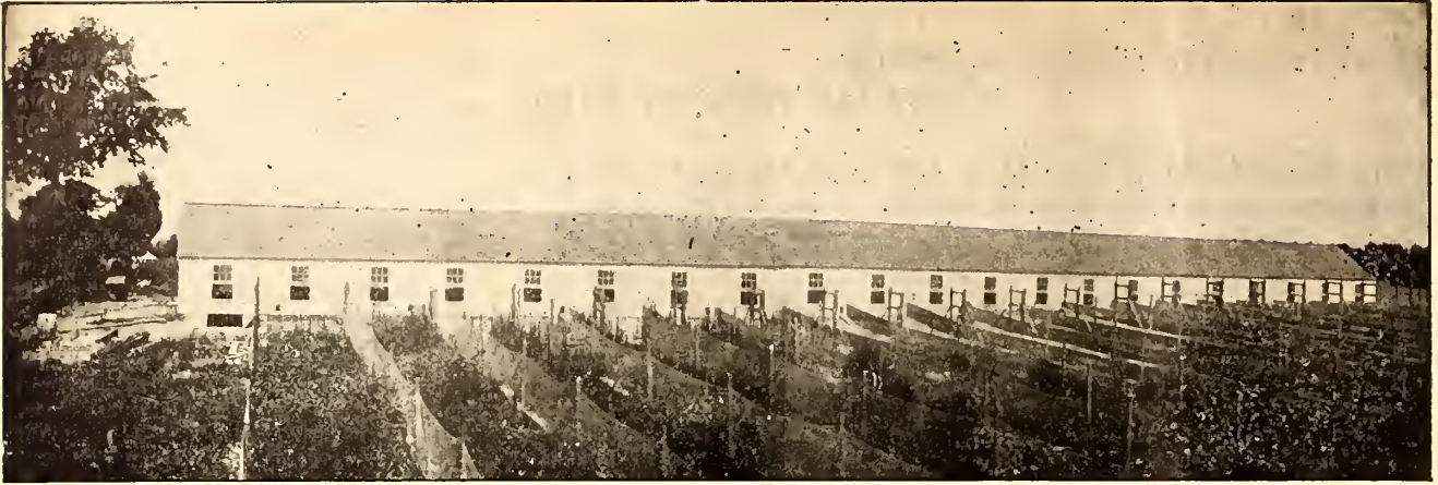
210x20 ft. Laying House on the Millville Poultry Farm, Millville, N. J. This building comprises 20 pens, 10x11½ ft; 40 pens, 5x5 ft; and a feed room, 10x20 ft.
