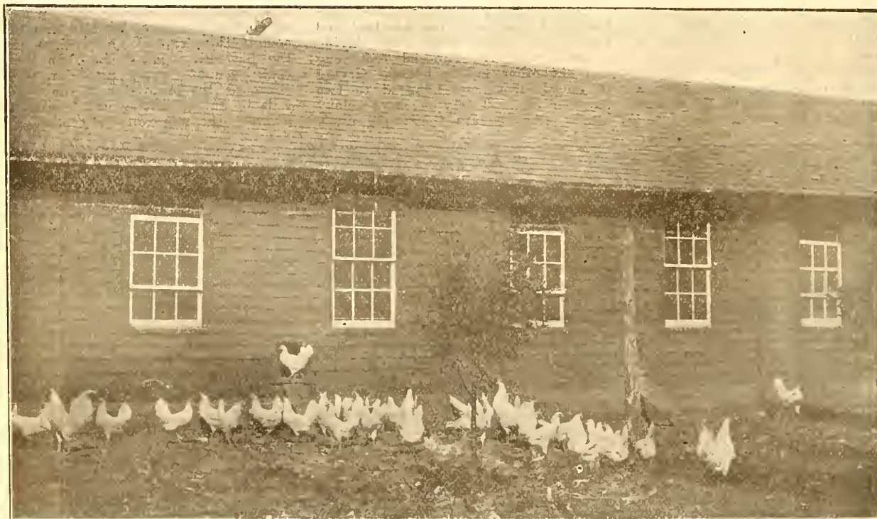
One of the laying houses at the White Leghorn Poultry Yards, Waterville, N. Y. Building is two hundred and fifty feet long by sixteen feet wide and accommodates five hundred layers.
