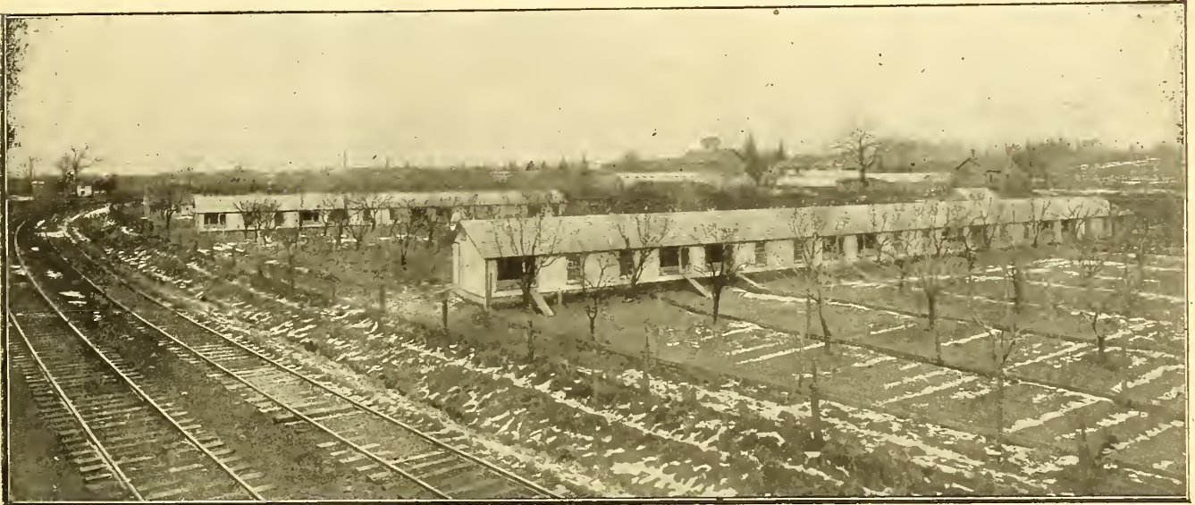
The "community" style of poultry house. The view shows a house 180 ft. long by 12 wide, divided into ten houses of 18 ft. each, sub-divided into scratching shed and laying and roosting room.
