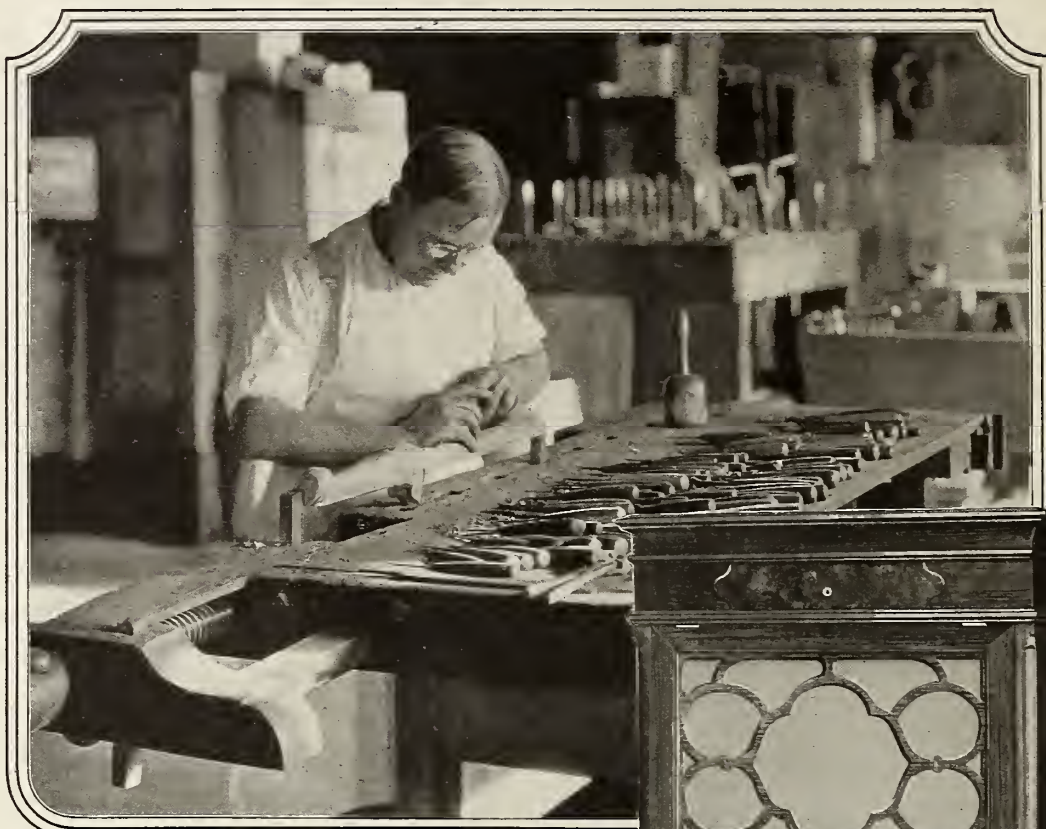
One of the hand carvers modeling the legs of a Cheney cabinet in the Georgian Period style
