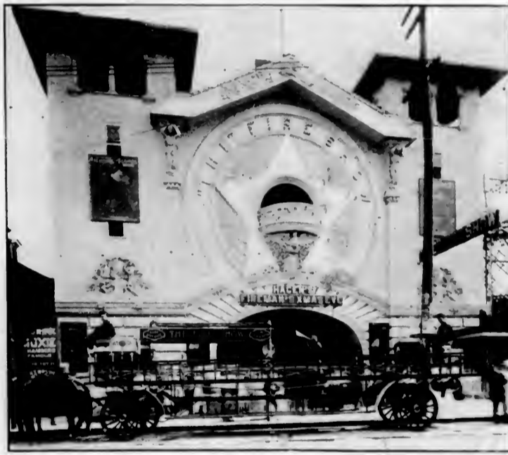
Front view of Claude Hagen's Fire Show in the old Galveston Flood Building at Coney Island, New York, showing the book-and-ladder ball-hoop.
