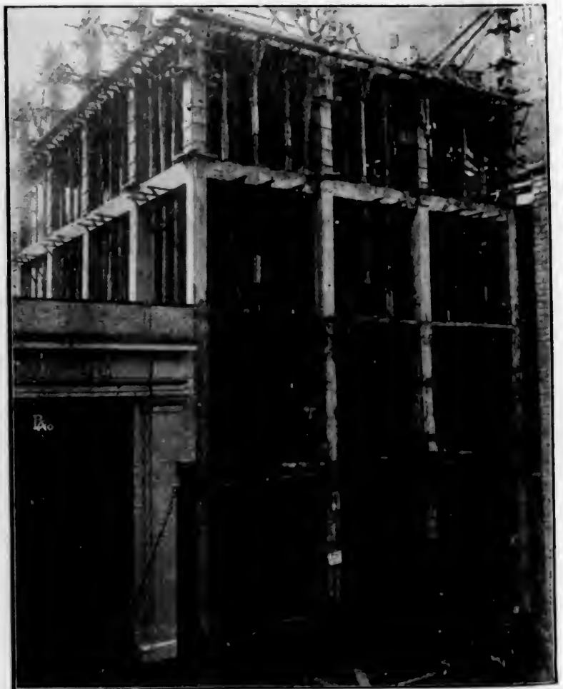
Four of the six stories of steel-concrete construction finished.
