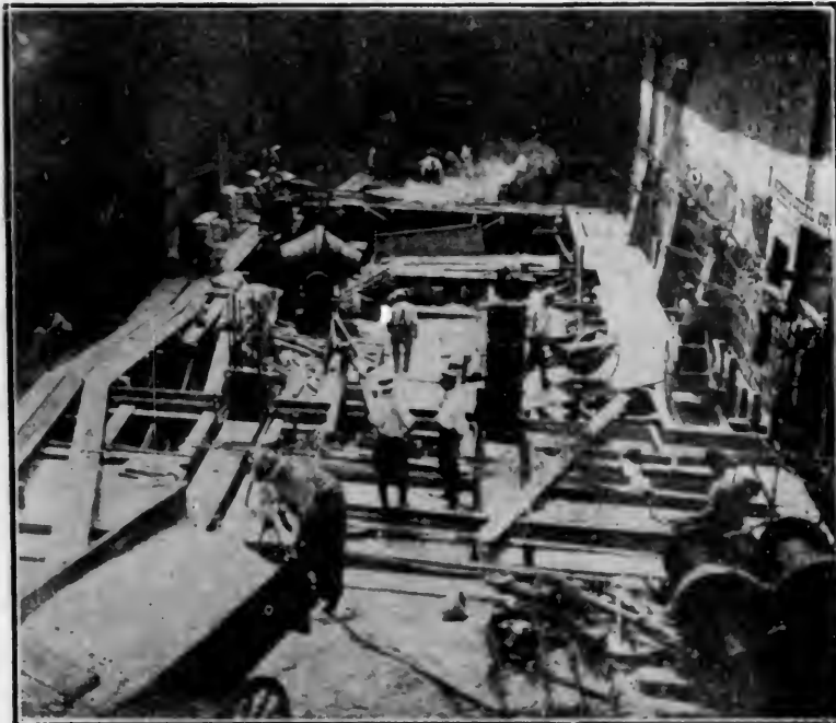
The first stage of construction.
