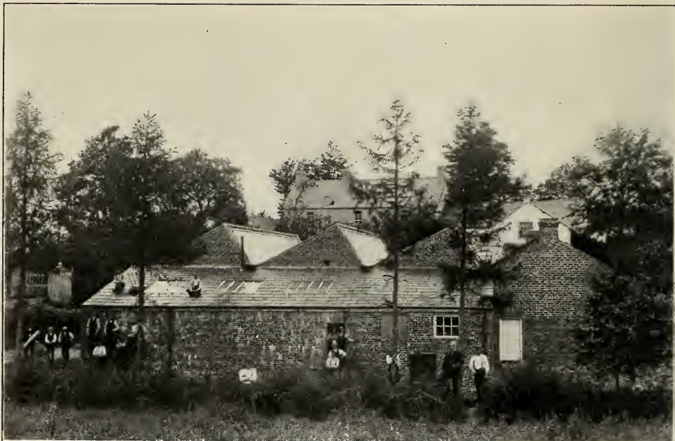
EXTERIOR OF A HAND-LOOM DAMASK FACTORY
