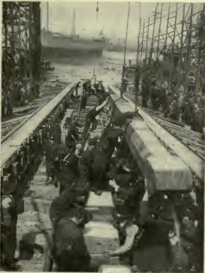
Fig. 29. Laying the Keel of Another Ship as Soon as the Accoma Left the Ways at the Foundation Company's Yard
