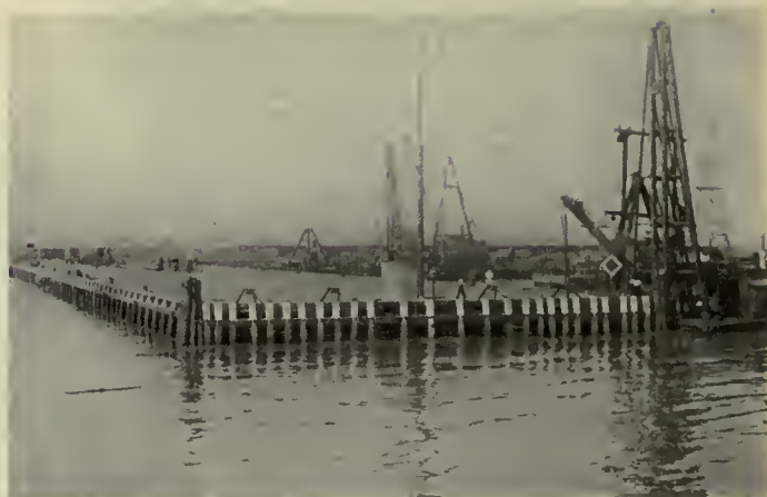
Thousands of Piles Are Driven Into the Marsh on Which to Build the Piers. The Picture on the Left Shows the Piling For Pier and That on the Right Shows Pier Completed and Ready For Use
