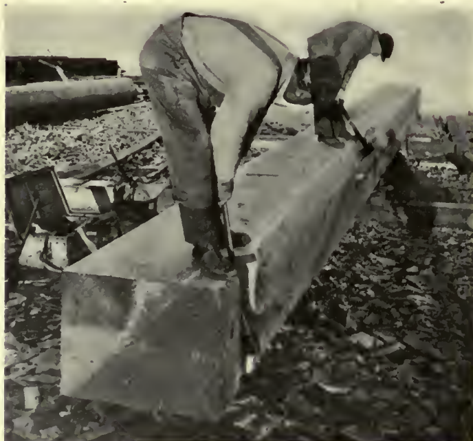
Fig. 124. Making a Spar
