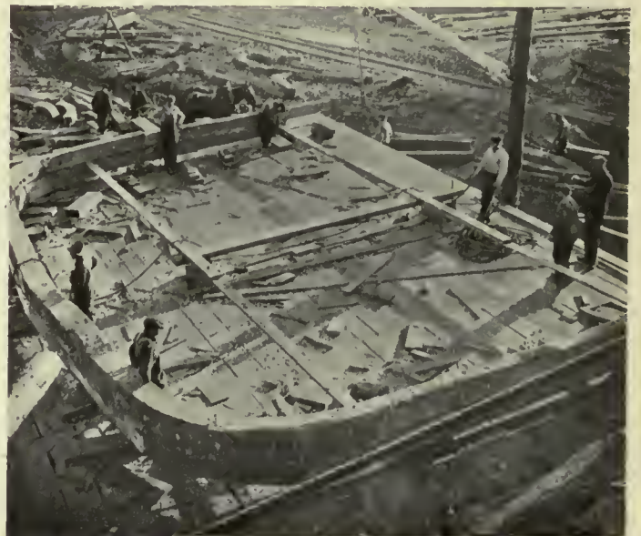
Fig. 75. Assembling a Midship Frame
