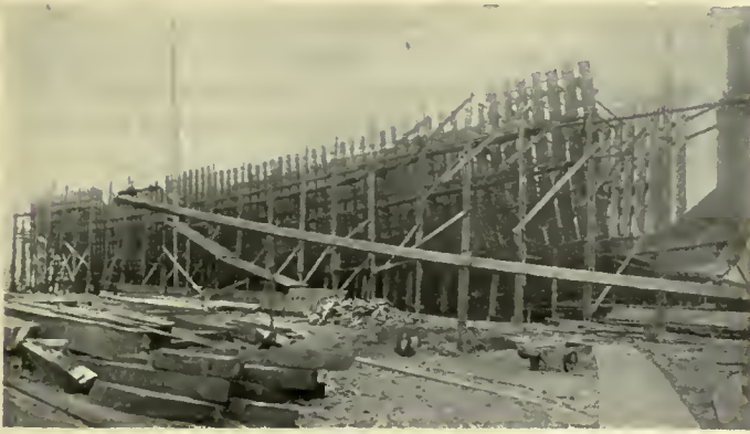
Fig. 79. Stem, Deadwood and Frame Set Up
