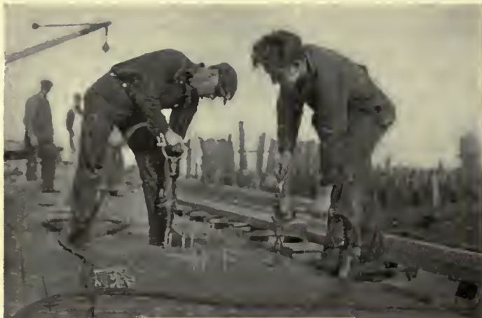
Fig. 97. The Pneumatic Hammer Driving Deck Spikes in Holes Which Have Been Drilled and Countersunk at the Same Operation by Another Little David. These Tools Make Short Work of Numerous Tasks
