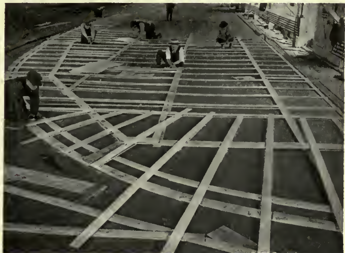
Fig. 73. Mould Loft Work
