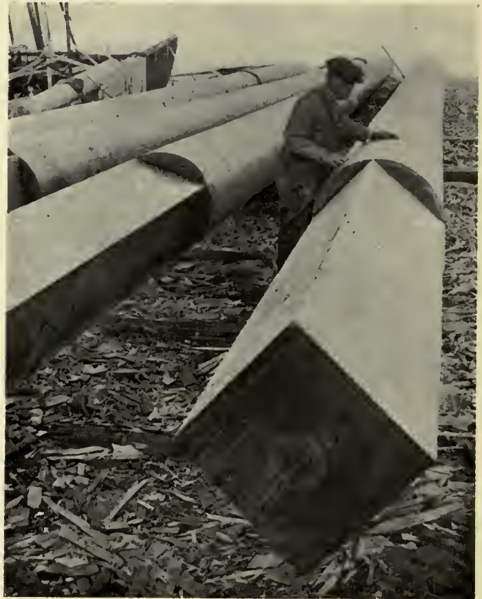
Fig. 125. Making a Spar
