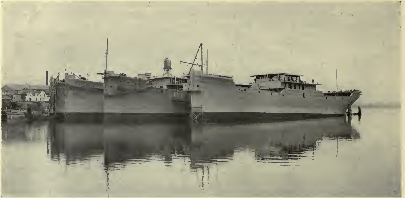
Fig. 143. Chibiahos, Roy H. Beattie, Milton and Haverhill, Four Ships Built by L. H. Shattuck, Inc., at Portsmouth, at the Dock Fitting Out With Rigging, Joiner Work, Etc.
