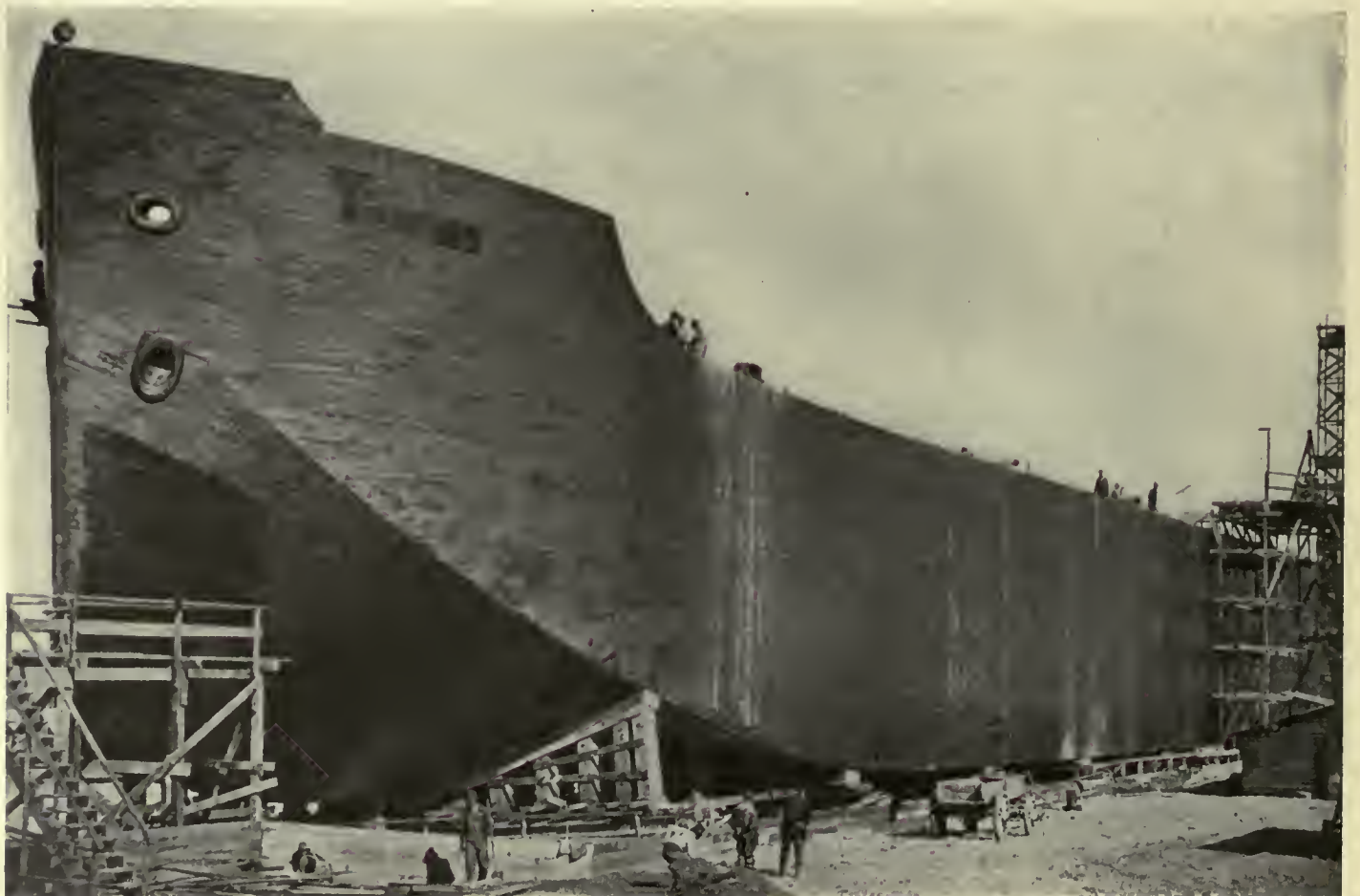
Fig. 150. Faith, 5,000-Ton Concrete Vessel, Launched 1918 From the San Francisco Shipbuilding Company's Yard at Redwood City, Cal.
