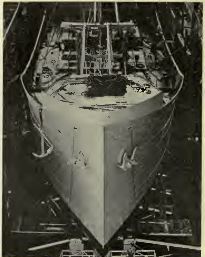
Fig. 157. Stockless Anchor in Place
