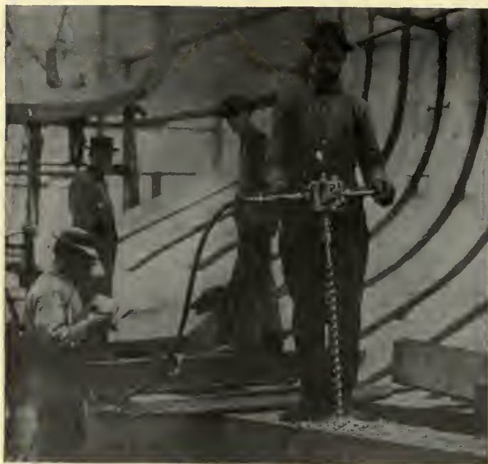
Fig. 81. The Little David Pneumatic Boring Machine Makes Light Work of the Deep Holes Required in the Giant Keelsons. The Operator Has to Have Only a Straight Eye and a Steady Hand, For His Task Is Not to Guide the Tool
