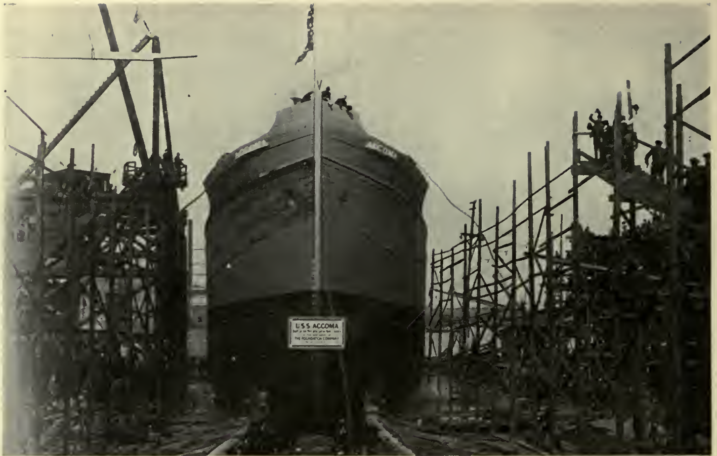
Accoma, Wooden Ship Built by the Foundation Company, Sliding Down the Ways Into the Passaic River
