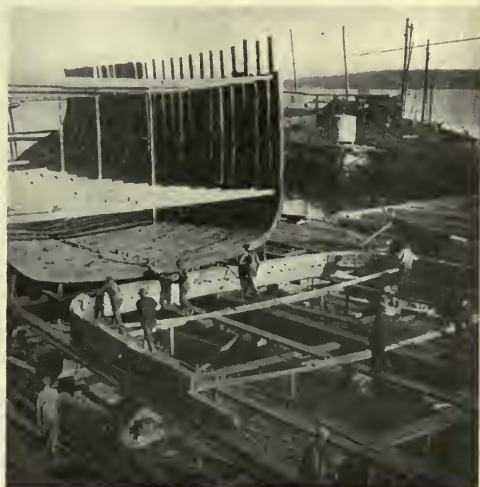
Fig. 76a. Erecting a Midship Frame
