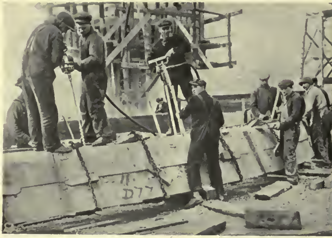
Fig. 74. Assembling a Frame
