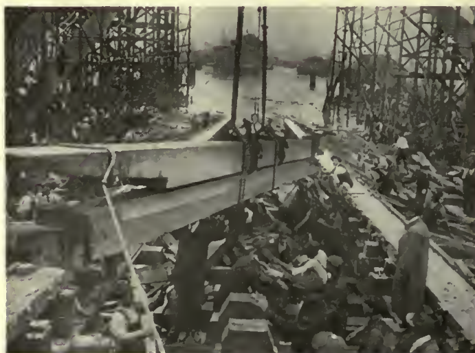
Fig. 31. As Soon as the Congaree Was Launched From the Foundation Company's Yard Workmen Laid the Keel For Another Vessel
