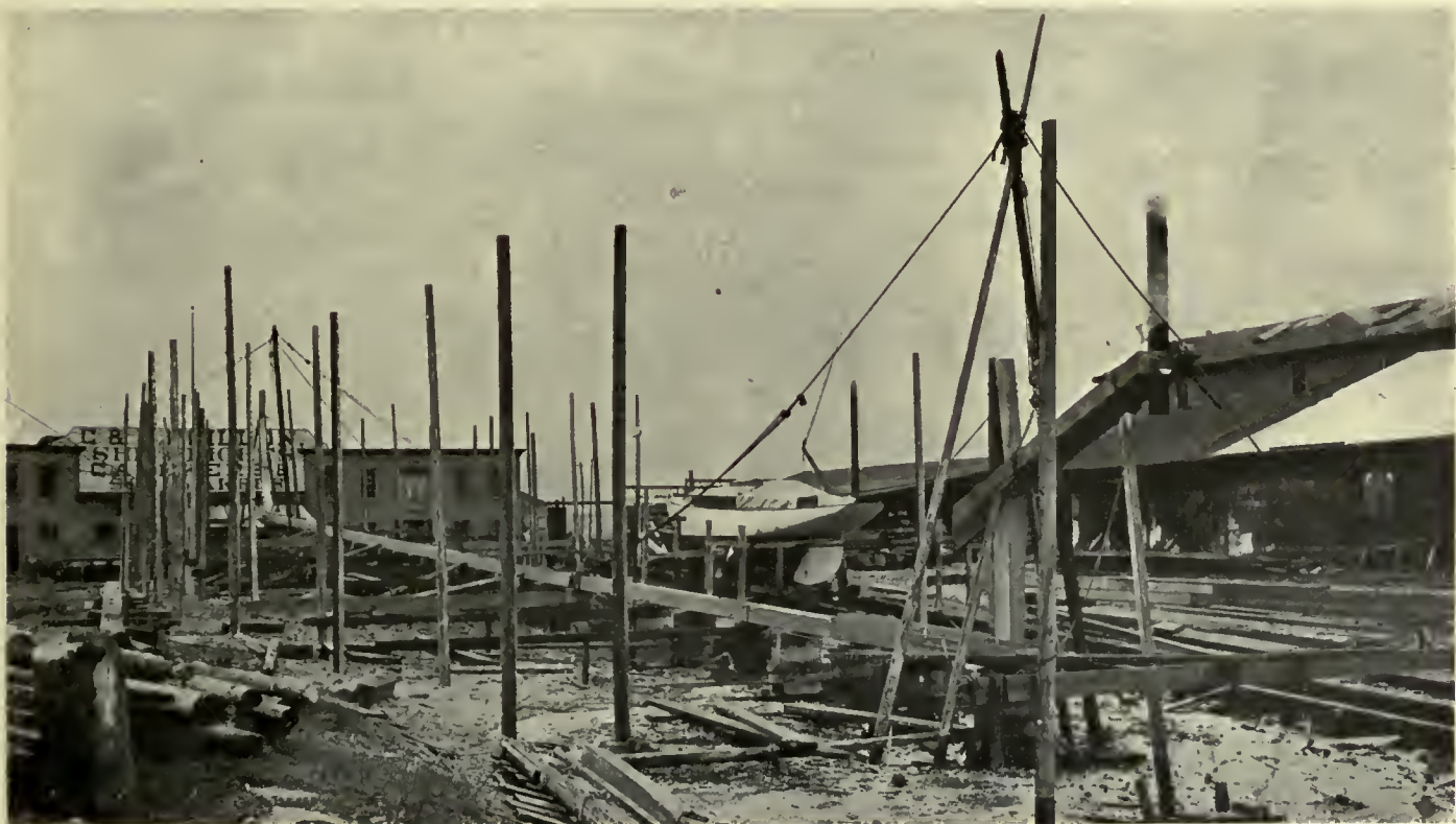
Fig. 82. Setting Up the Stern
