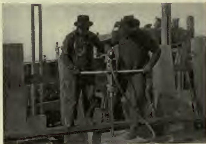
Fig. 81a. The Pneumatic Drift Bolt Driver Hammering Home a Long 1¼-In. Bolt Through a Deck Beam and Its Supporting Sturdy Sill. The Bolt Disappears Into Its Hole With Astonishing Rapidity
