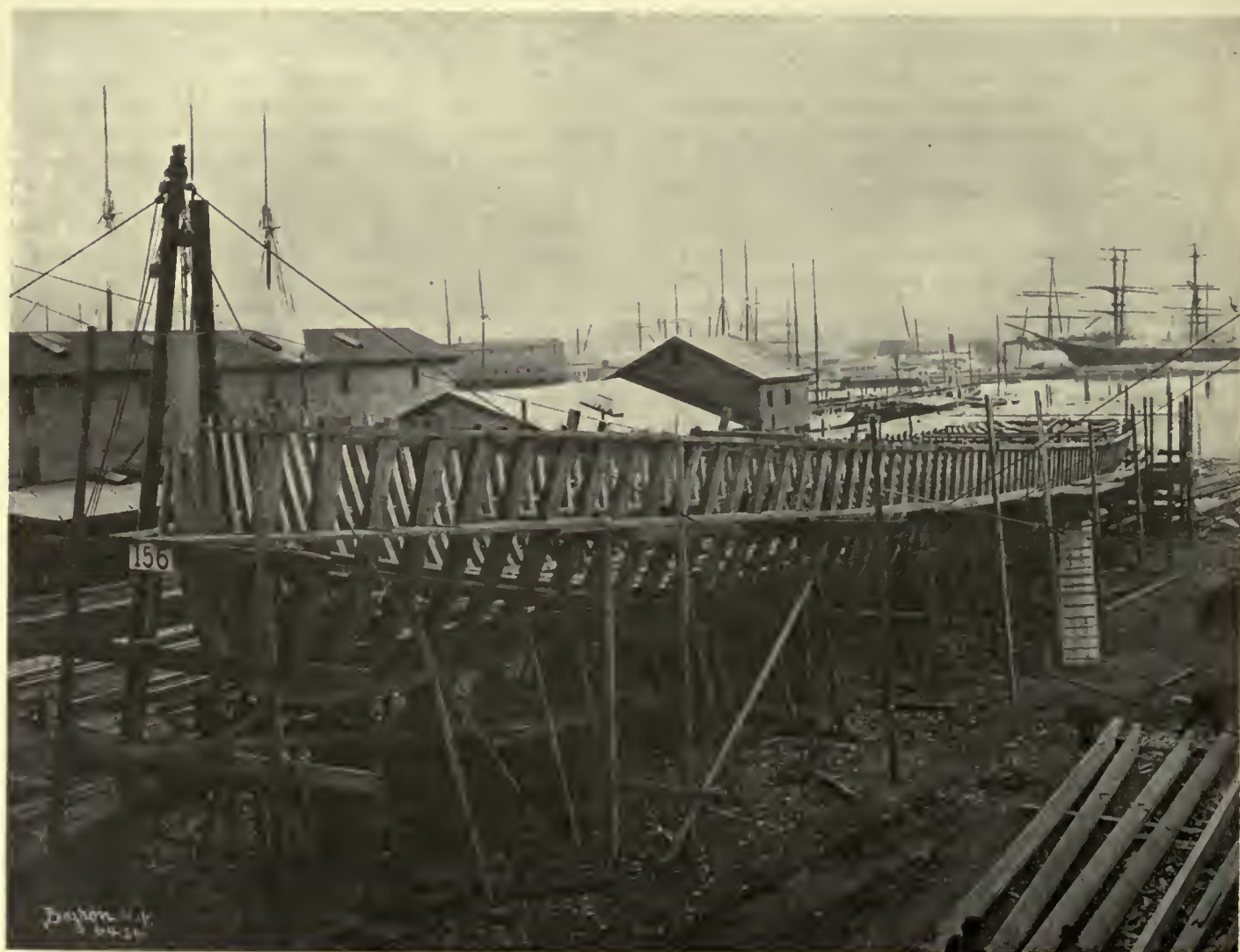
Fig. 90. Framed Ready For Sheer
