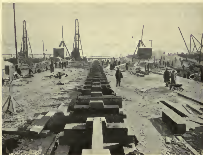
Keel Blocks Being Laid
