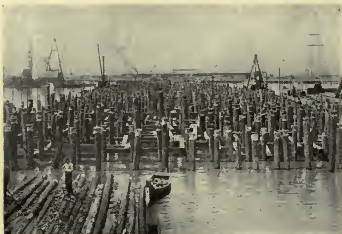
Thousands of Piles Are Driven Into the Marsh on Which to Build the Piers. The Picture on the Left Shows the Piling For Pier and That on the Right Shows Pier Completed and Ready For Use
