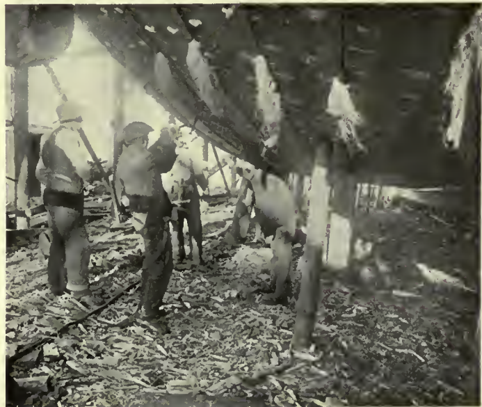
Fig. 93. Caulking Bottom Planking
