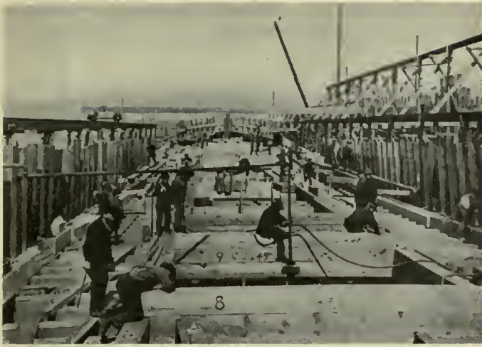
Fig. 53. Deck Framing and Waterways
