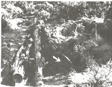
Figure 87. View of the historic structure foundation at 5RB399, located on tract 4. Cast iron stove (arrow) was half-buried in the fill.
