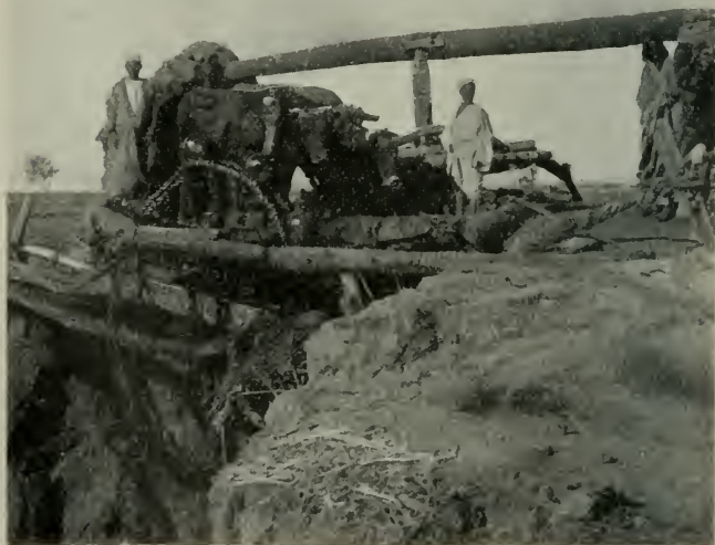
A modern water-wheel worked by oxen.
