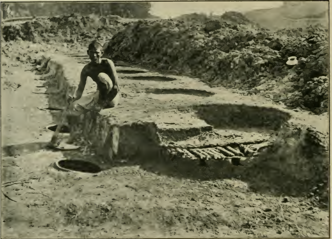
FIG. 3. Percolators for Extracting Indian Crude Saltpetre.
