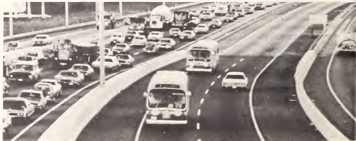
Shirley Highway's (I-95) separated, exclusive bus and carpool lanes cut substantial time from commuting trips between Washington, D.C. and its northern Virginia suburbs.
