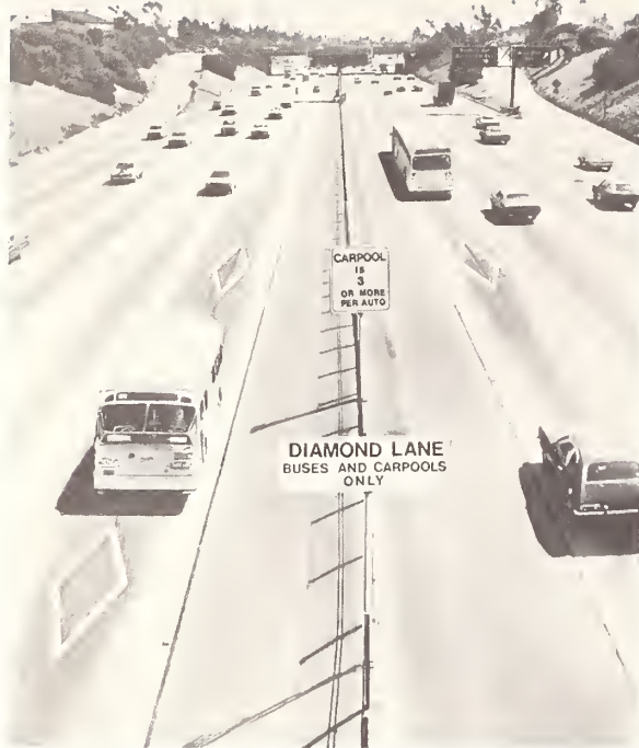
"Diamond Lanes" provide non-separated bus and carpool lanes on the Santa Monica Freeway near Los Angeles, California.
