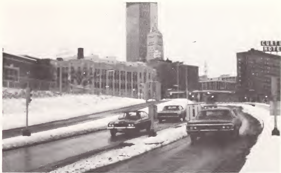
Metered freeway ramps combined with bus signal preemption controls are expected to speed traffic flow in Minneapolis (I-35W).
