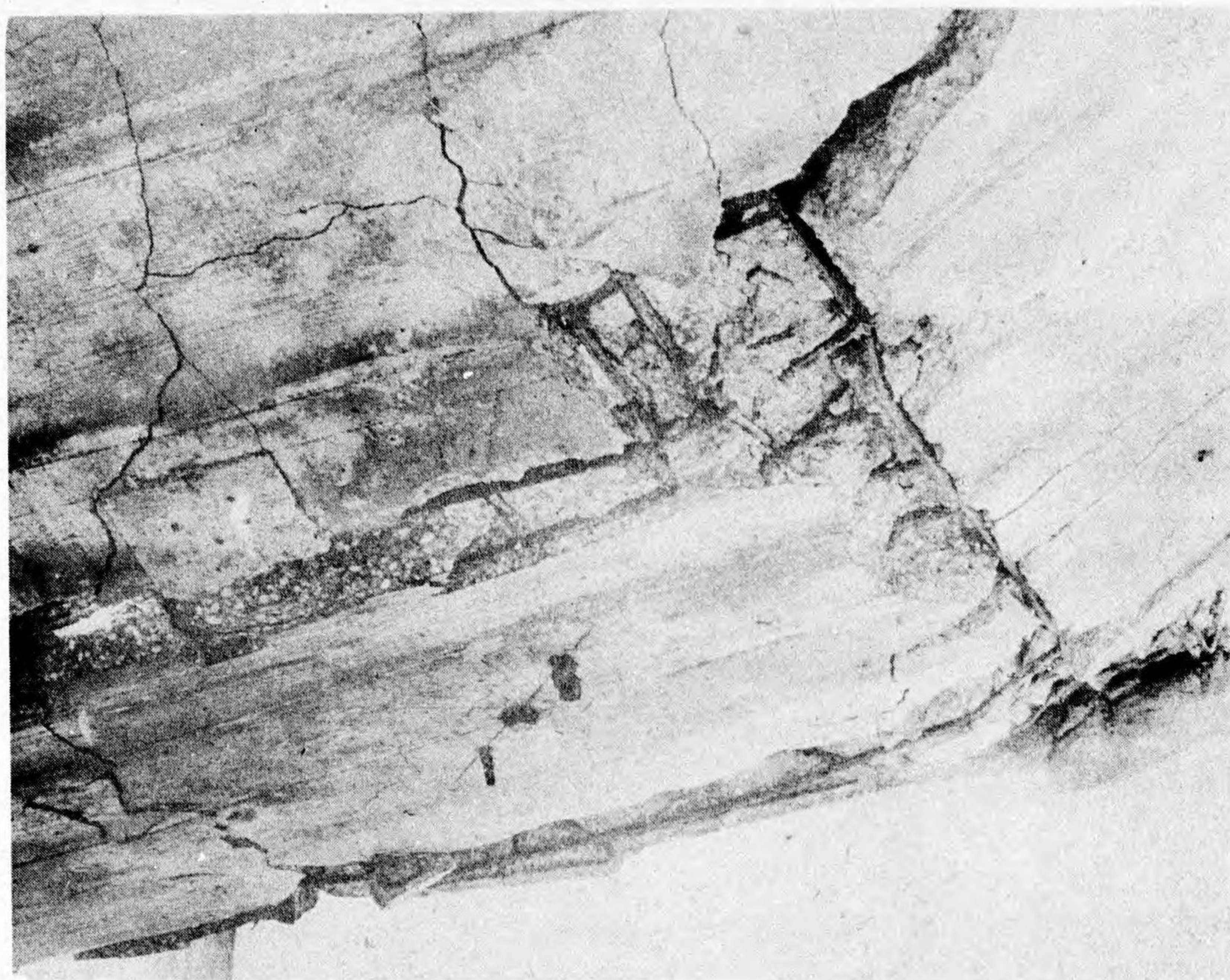
Fig. 10. Under side of first floor looking upward, after detonation of \frac{1}{2} lb of TNT. Only one bar failed in tension.
