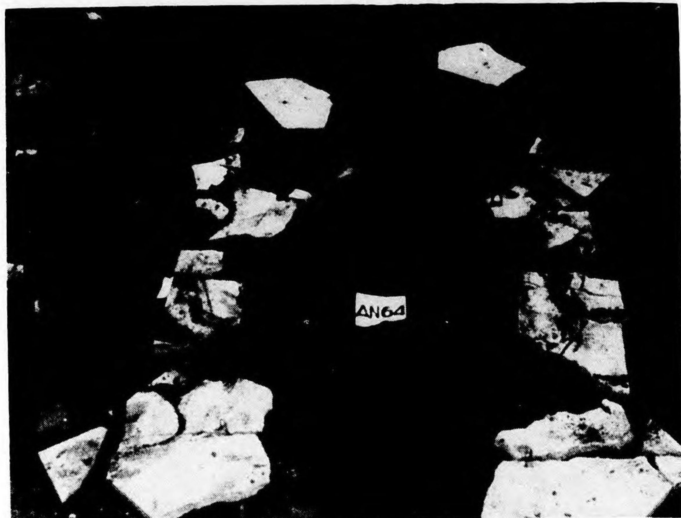
Fig. 1. A damage: Slab is completely destroyed and only a few isolated pieces of concrete remain.
