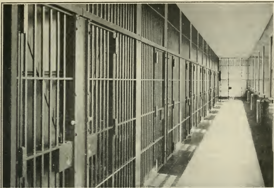
INDUSTRIAL FARM, BURWASH. TYPICAL CELL CORRIDOR.
