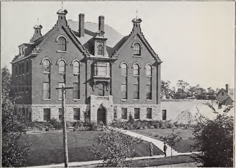
FIG. 2.—MINNESOTA COLLEGE AND STATION—HORTICULTURAL BUILDING.
