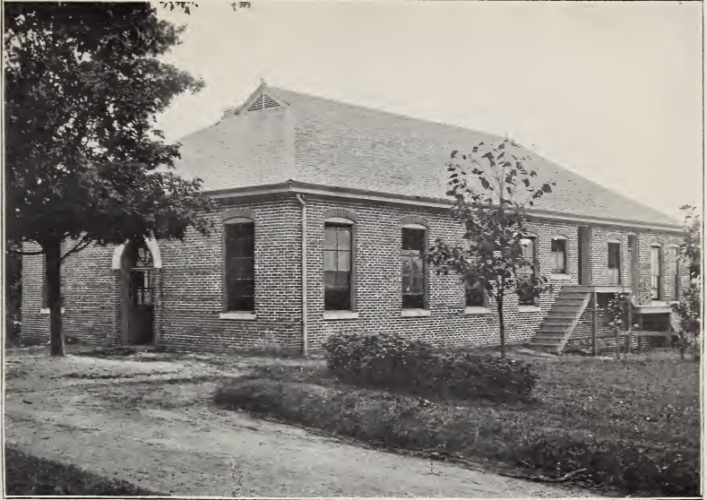
FIG. 1.—TENNESSEE STATION—DAIRY HALL.
