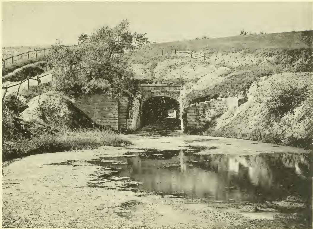
OLDEST TUNNEL IN THE UNITED STATES, BUILT 1822-3 FOR UNION CANAL—739 FEET LONG.
