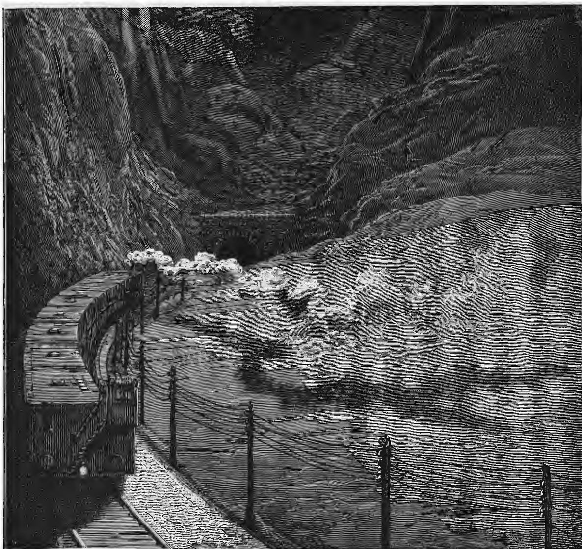
GORGES OF PANCORBO : THE TUNNEL.
