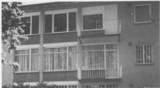
In the Bonn housing complex, first and second floors have the original steel-framed
