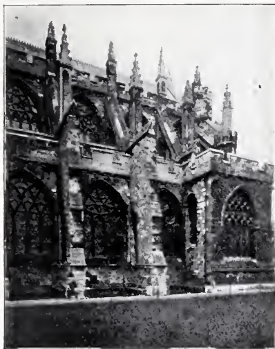
NORTH SIDE OF NAVE ST. PETER'S CATHEDRAL, EXETER.
