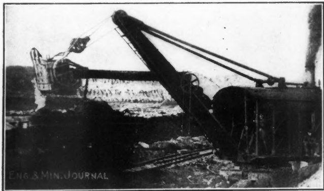
FIG. 3. SHOVEL EMPTYING LOAD INTO A FLAT CAR
