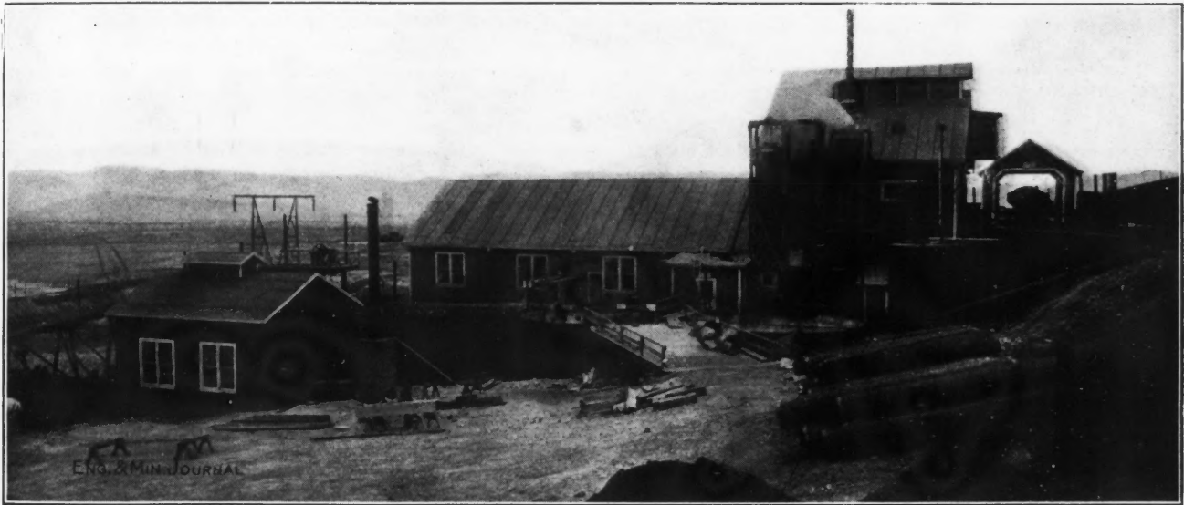
THE ANACONDA COMPANY'S EXPERIMENTAL LEACHING PLANT FOR COPPER ORES
