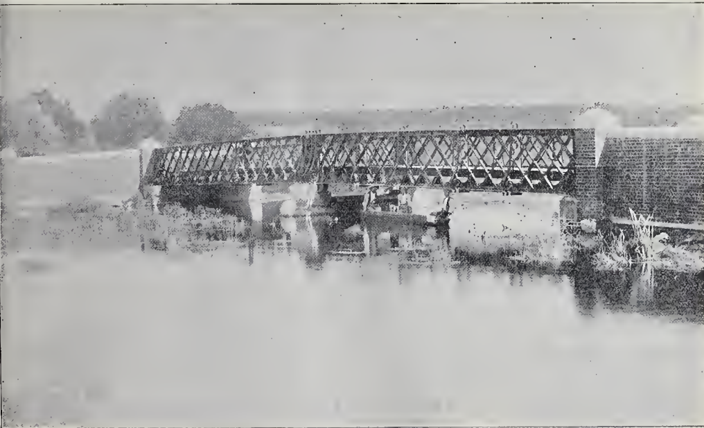
Breamore Bridge. Mr. W. J. Taylor, Engineer.
