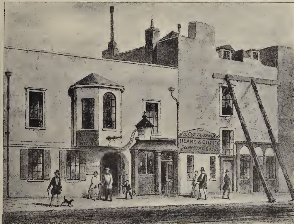
THE GUN TAVERN; pulled down in 1857; site now partly occupied by Buckingham Palace Hotel
