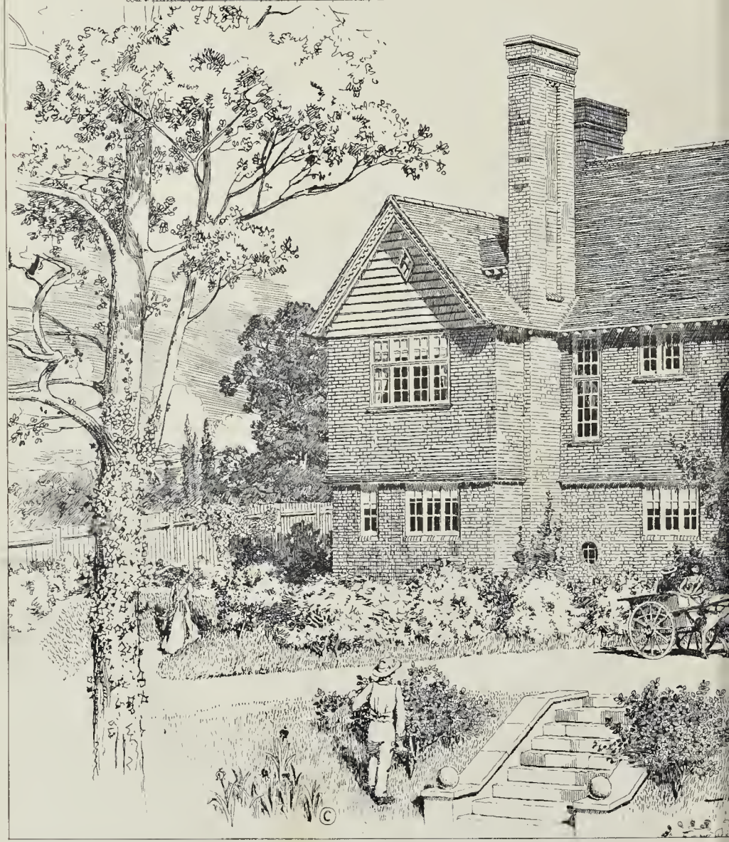
HOUSE AT CHISLEHURST: EXTERIOR
