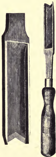
FIG. 8.—The "Michie-Golledge" Tapping Tool.
