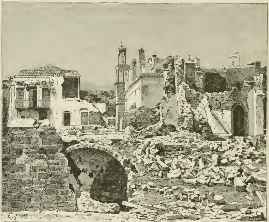
Fig. 136.—CHIO—VIEW TAKEN AFTER THE EARTHQUAKE OF 1881.
