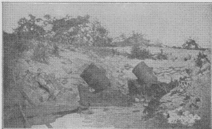
Battery Kirby: Twenty-eight-inch Seacoast Mortars against Sumter.
