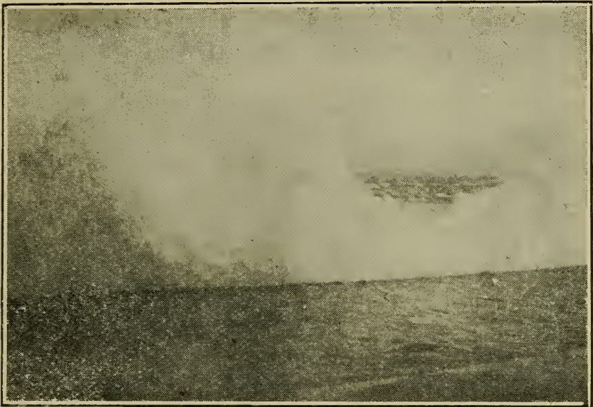
A high wave breaking over the sea wall at St. Malo, France, which is built upon a rocky island in the English Channel and is protected by the wonderful sea wall, shown in the foreground.
