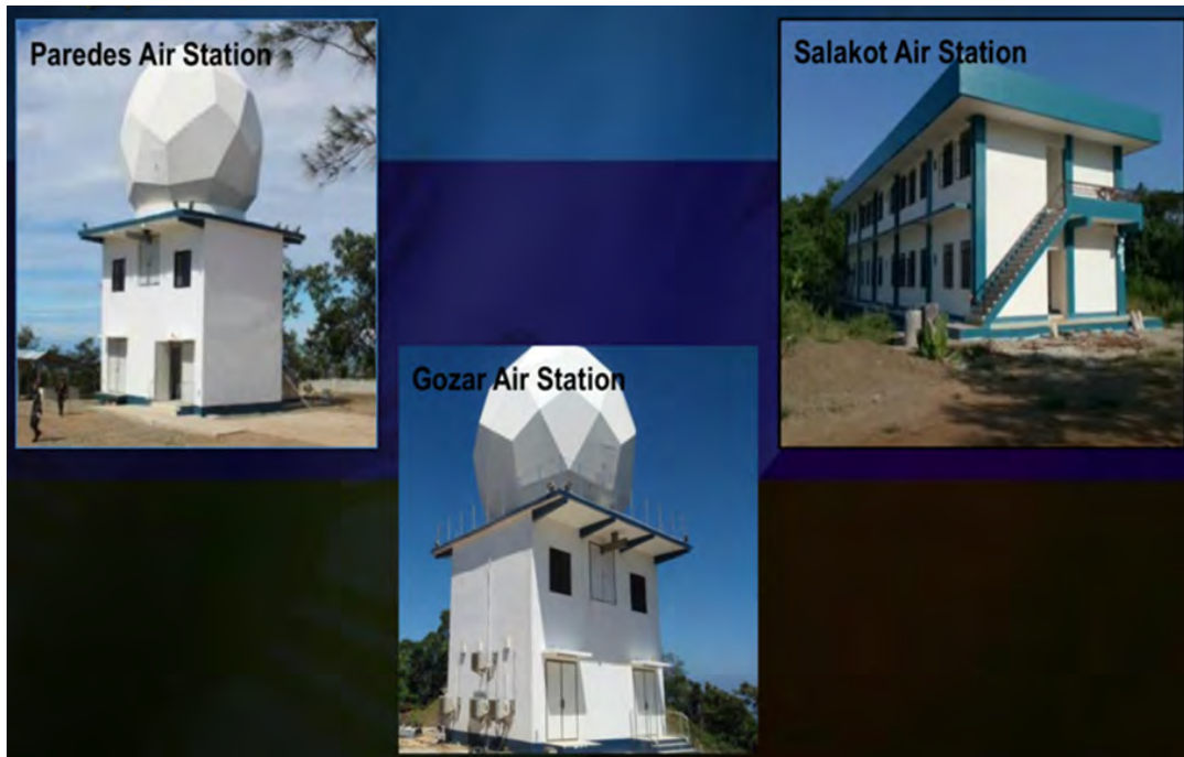
In photo: Air Surveillance Radar installed at Paredes and Gozar Air Stations. Installation in the Mt. Salakot Air Station is ongoing.
