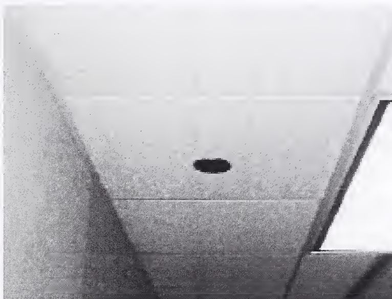
Figure 3–7. Typical concealed pendent sprinkler.
