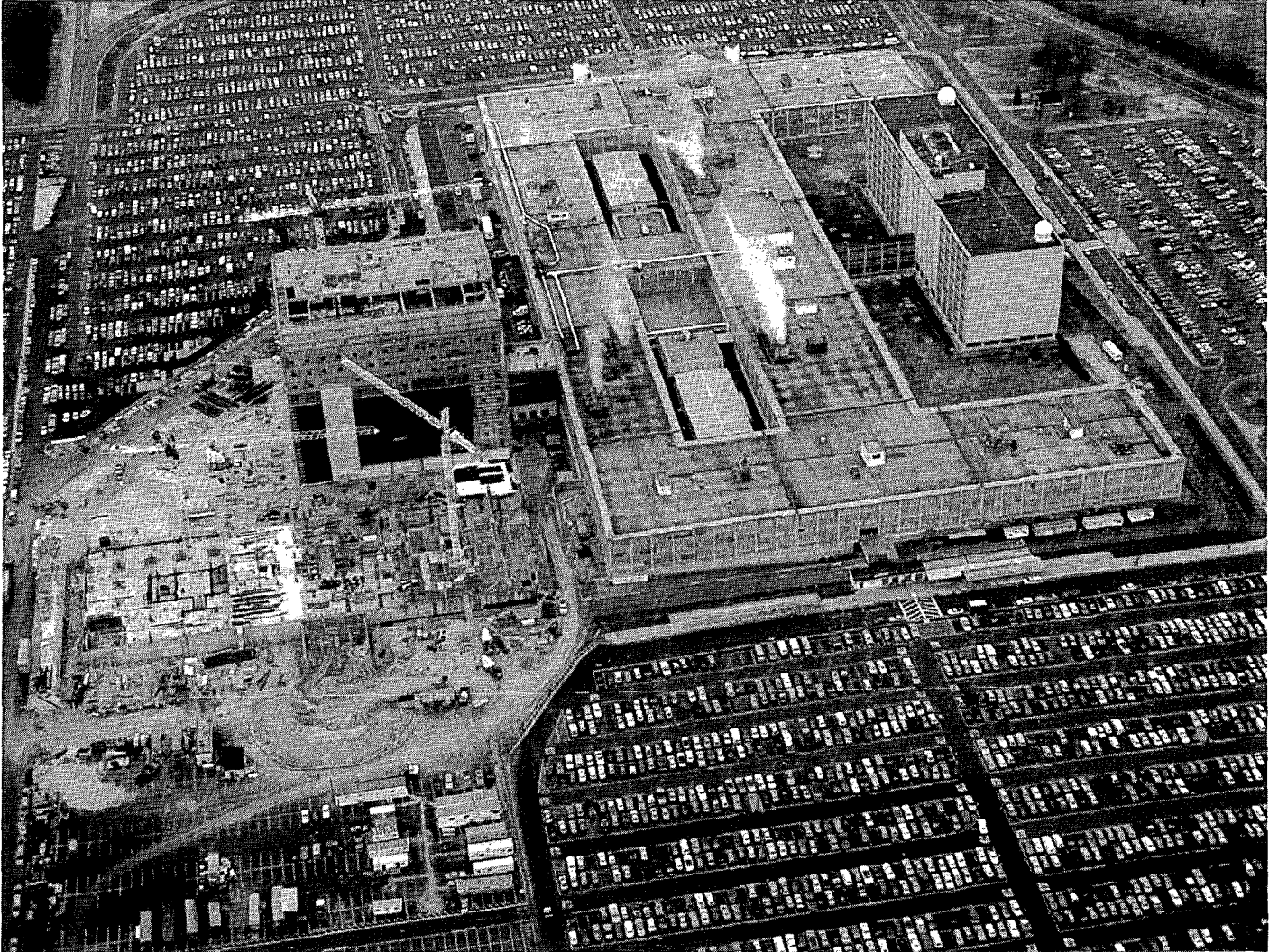
(U) Construction of Ops 2A
