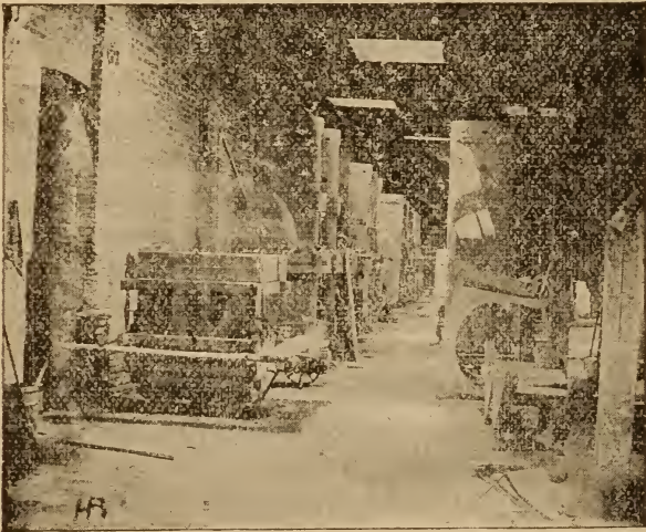
Molding-room of Gas-retort Works.
