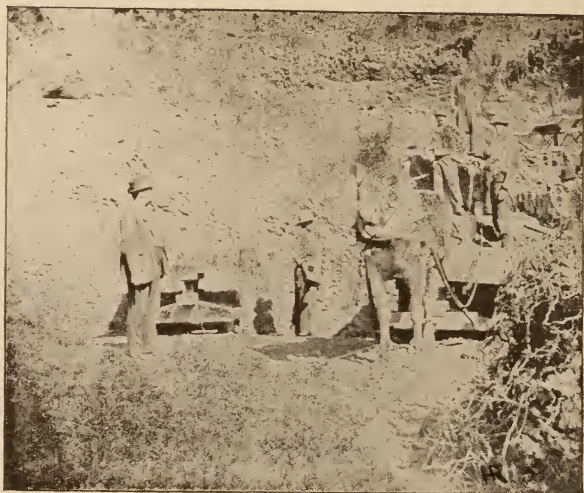
Loading clay on cars.
