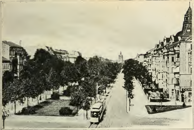
SPACIOUS STREET CONSTRUCTION, CHARLOTTENBURG.
