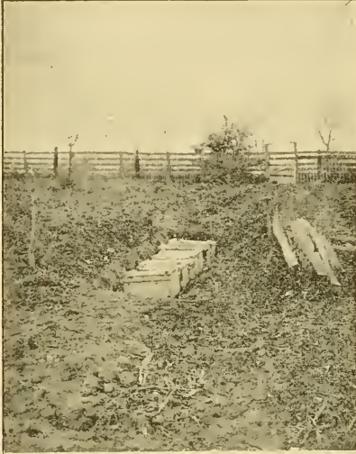
READY FOR THE RAILS.
