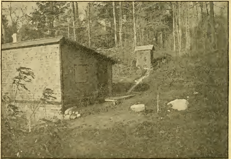
FIG. 1.—FRONT VIEW OF "CABIN IN THE WOODS."
