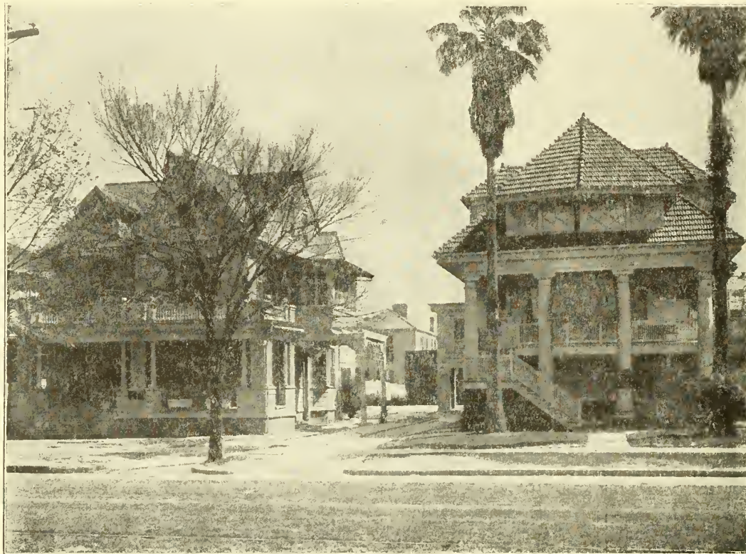
Some of the Clinic Buildings
