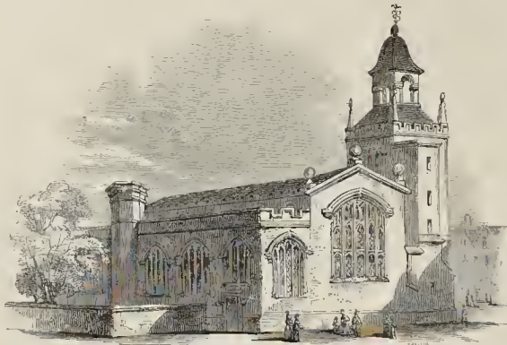
CHURCH OF ST. ANDREW UNDER SHAFT.
