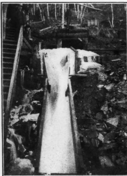
WATER COMING OUT OF NORTH END TUNNEL SHOWING FOAM CAUSED BY GAS
