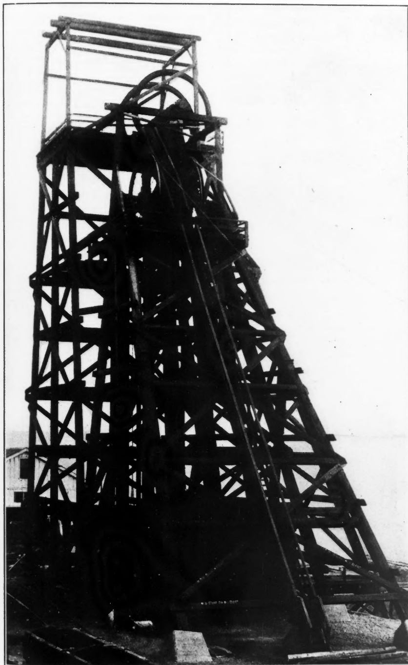
FIG. 10. BACK VIEW OF EAST BROOKSIDE COAL SHAFT HEAD FRAME
