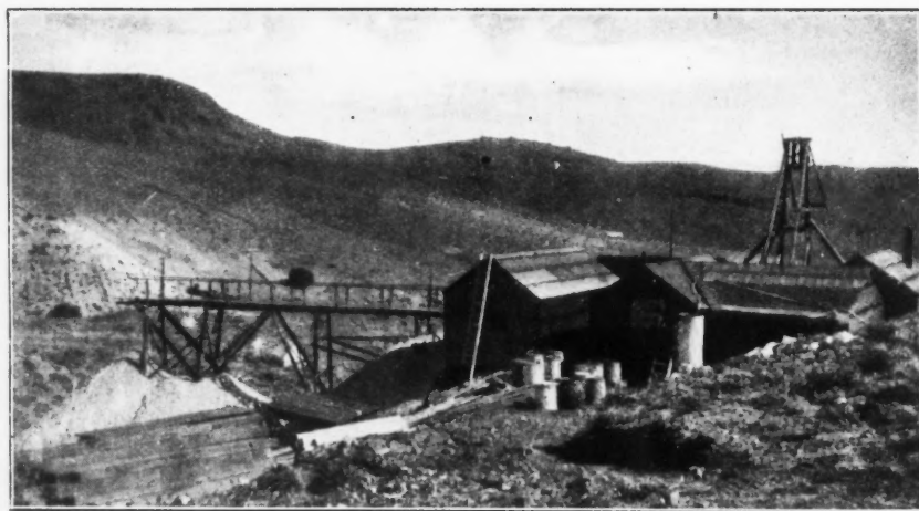
SEVEN TROUGHS MINE, HUMBOLDT COUNTY, NEVADA
