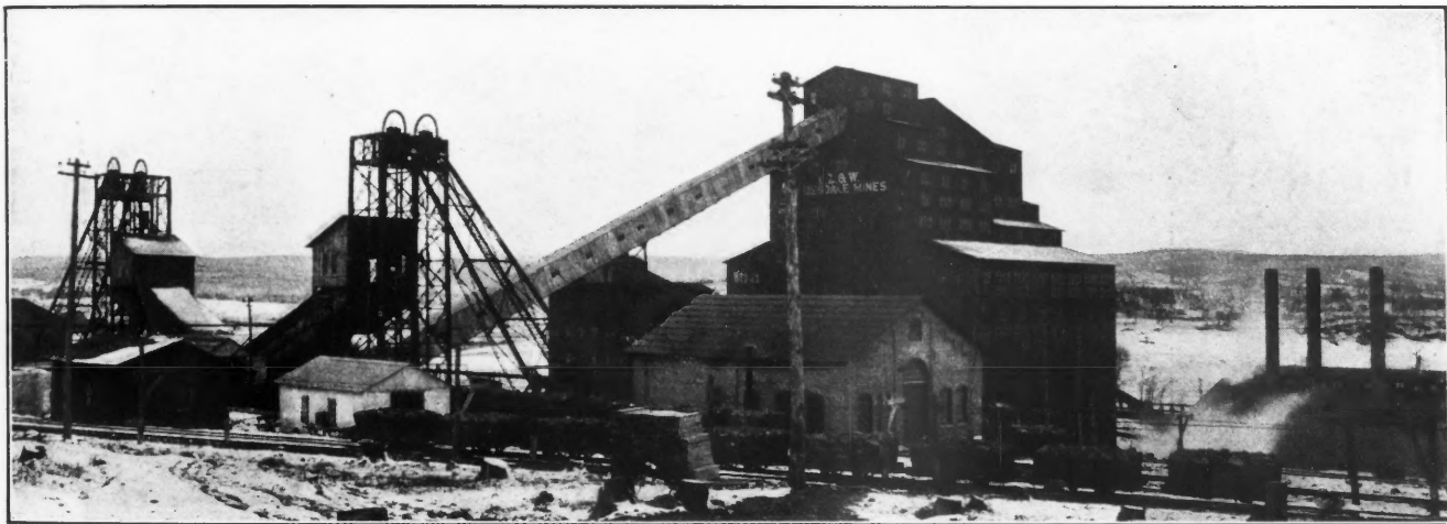
FIG. 1. HOISTING PLANT AND CONVEYER LINE TO BREAKER AT TRUESDALE COLLIERY, NEAR NANTICOKE, PENN.
