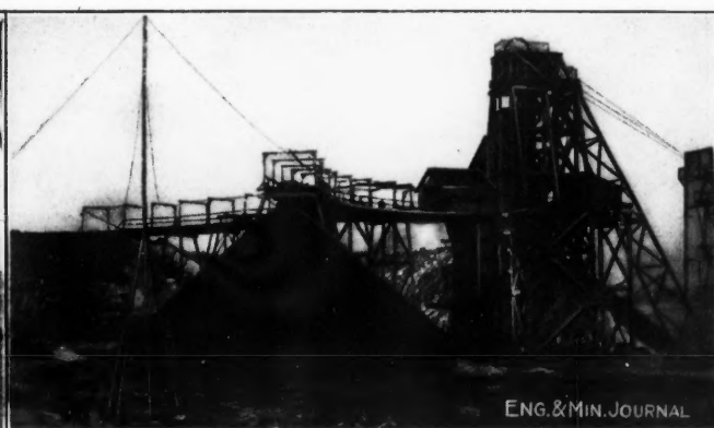
FIG. 8. MARY CHARLOTTE STOCKPILE. NOTE GUYED MAST TO SUPPORT THE SURPLUS TROLLEY WIRE
