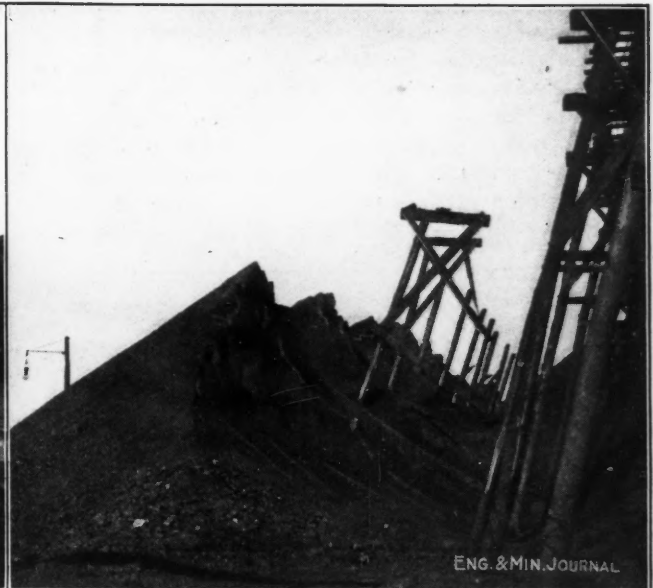
FIG. 4. PARTLY LOADED OLD STOCKPILE OF PENN COMPANY, OLD BENTS STILL SHOWING AND NEW TRESTLE ON RIGHT
