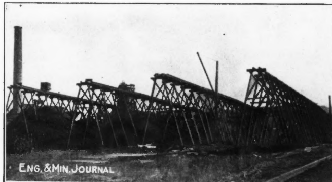
FIG. 5. FOUR PARALLEL TRESTLES WITH ENDLESS ROPE HAULAGE, AT CASPIAN MINE
