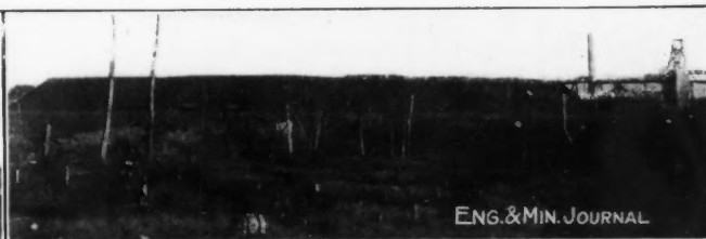
FIG. 2. THE COMPLETED STOCKPILE OF THE WHITESIDE MINE. THE BENTS NEAR THE HEADFRAME ARE STEEL
