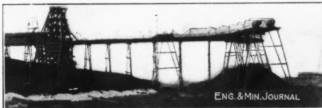
FIG. 1. BEGINNING OF STOCKPILE AT CHISHOLM MINE. NOTE BRANCHING TRESTLE AND TAIL-TRACK HOUSING
