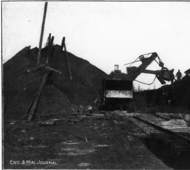
FIG. 3. STEAM SHOVEL RELOADING STOCKPILE AT WOODBRIDGE MINE. NOTE OLD TIMBERS IN THE ORE
