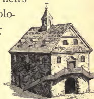
COLONIAL COURT-HOUSE, PHILADELPHIA. BUILT 1707.
