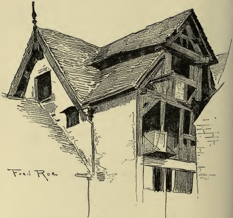
Timber-built House, Shrewsbury
