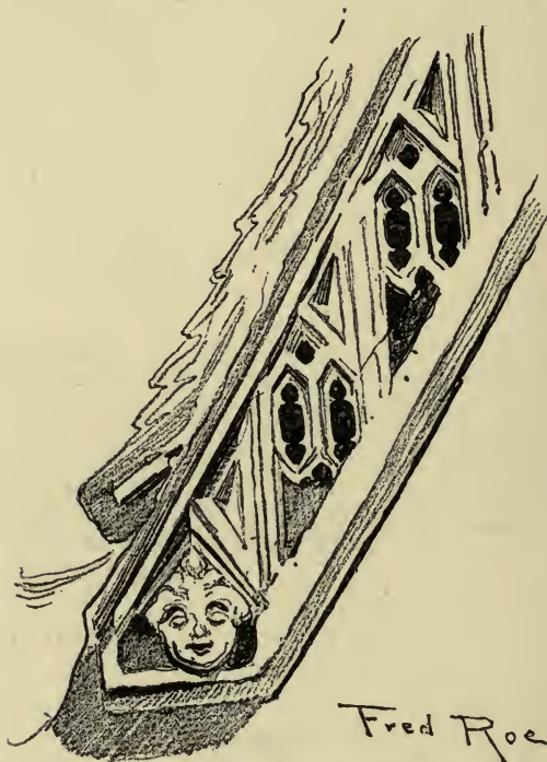
Detail of Fifteenth-century Barge-board, Burford, Oxon.
