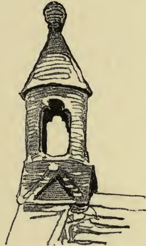
Gothic Chimney, Norton St. Philip, Somerset
