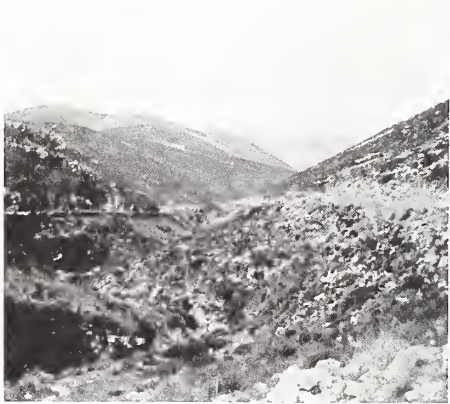
FIG. 14.—The new road and the old between Fondi and Itri, looking toward Fondi.
