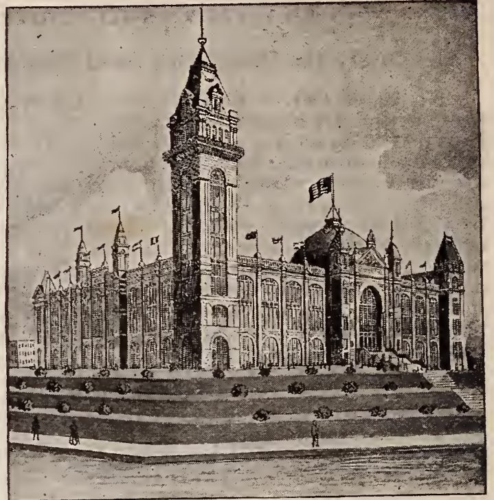
Minneapolis Exposition Building
