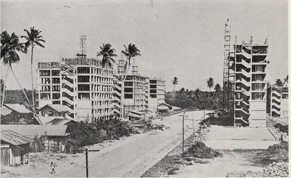
10-storey block of flats in MacPherson Road (South) Estate under construction.
