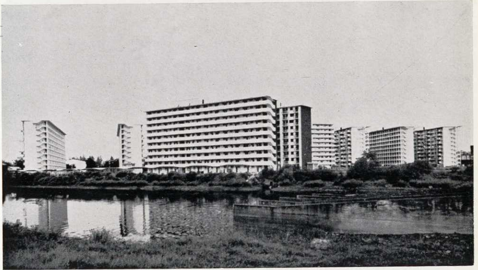
Panoramic view of Tanjong Rhu/Fort Road Housing Estate.
