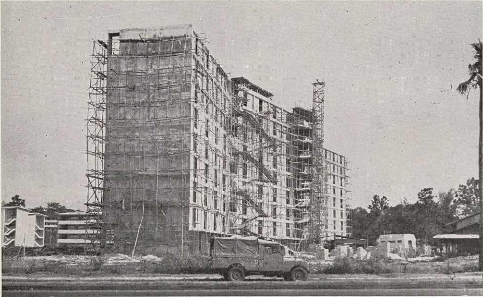
9-storey 3-room flats under construction in Clarence Lane, Queenstown.
