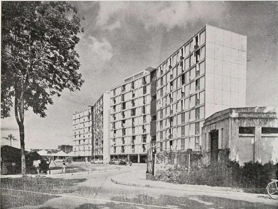
Another view of the 9-storey flats in Clarence Lane after completion. It contains 8 shops and 64 3-room flats.
