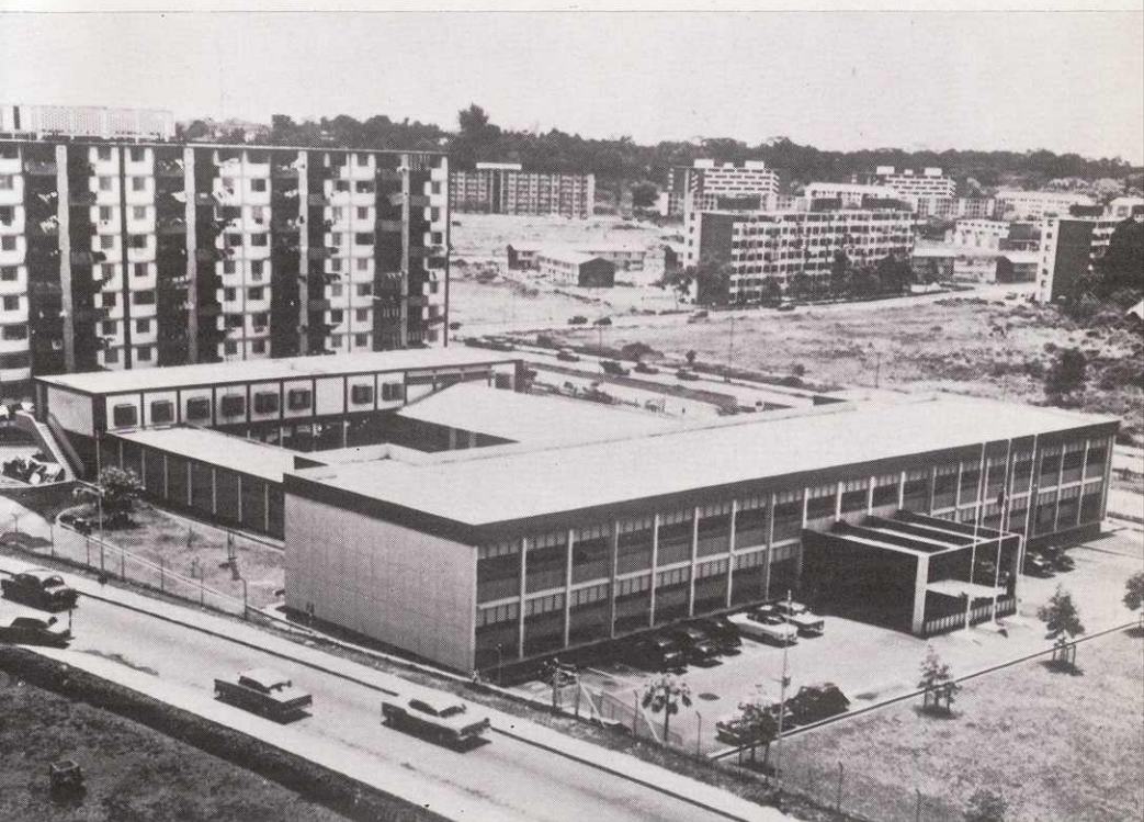
Aerial view of Queenstown Police Station built by the Housing Board in Neighbourhood IV for the Malaysian Police Force.
