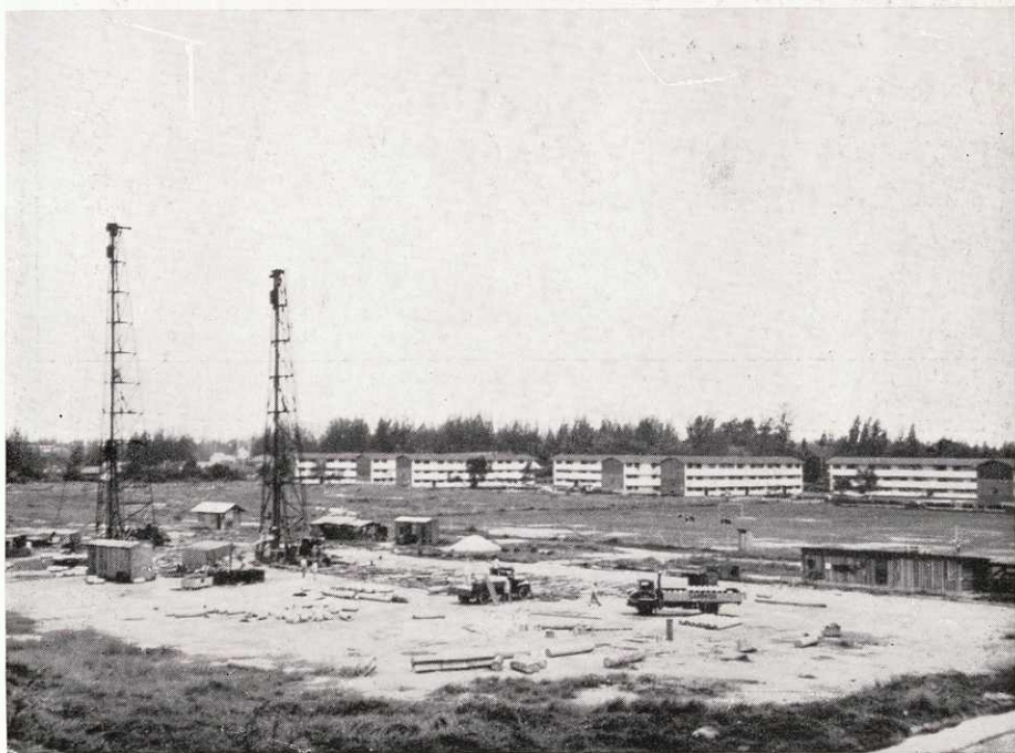
Piling operations at the Kallang Estate
