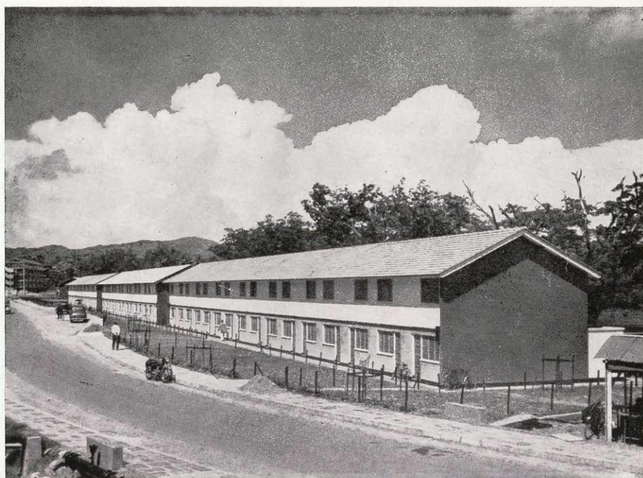
Kampong Tiong Bahru Fire Site Phase I. Comprising 2 storey 3 room terrace houses completed in 1960
