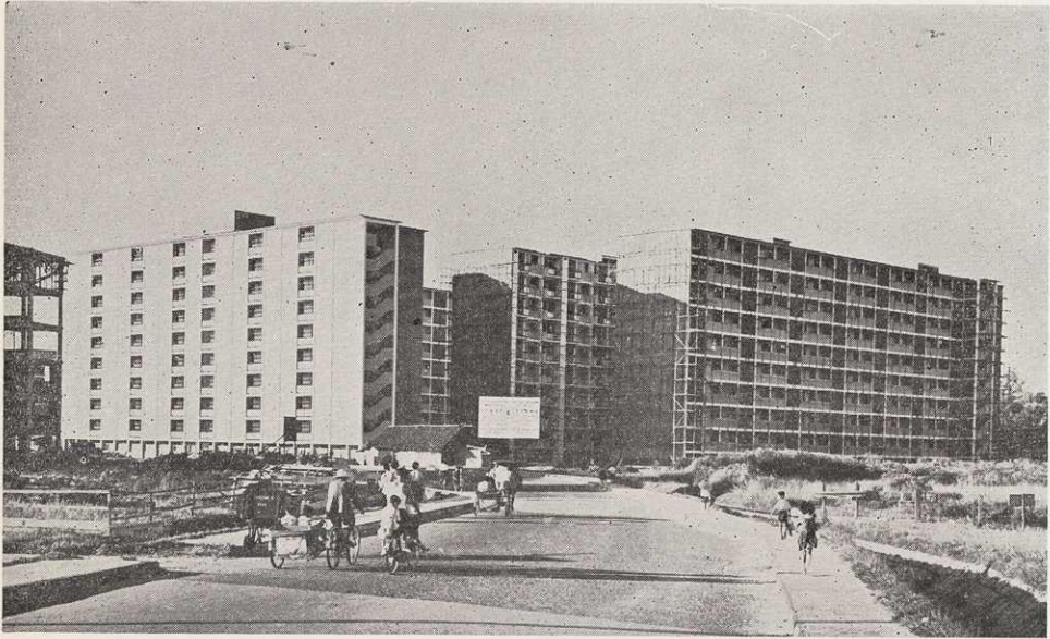
10-storey block of flats in St. Michael's Estate under construction.
