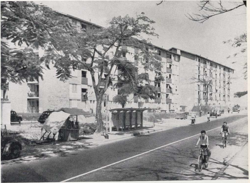
Bukit Ho Swee Estate — Blocks of 6-Storey one room flats built on site of fire which occurred in May, 1961.
