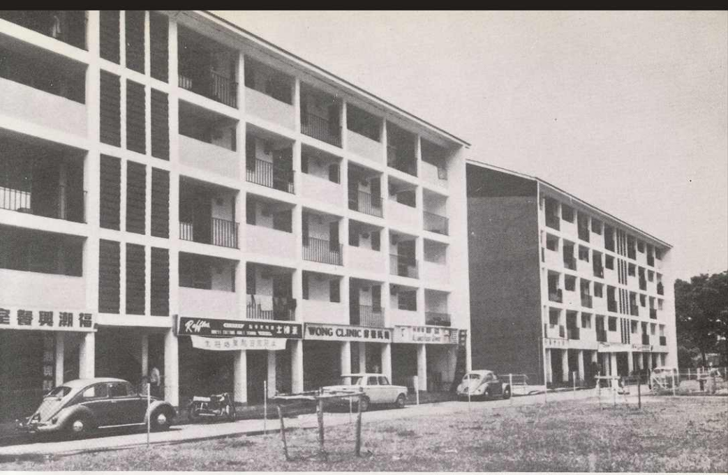
Siglap Fire Site Housing Estate. View showing two blocks of 5-storey 2-room flats with shops on ground floor.
