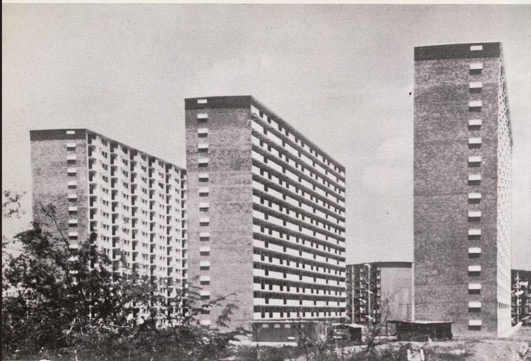
An impressive view of three 16-storey blocks of flats in Queenstown Neighbourhood III. These flats are offered for sale to the public. In the background are completed 10-storey blocks of flats.
