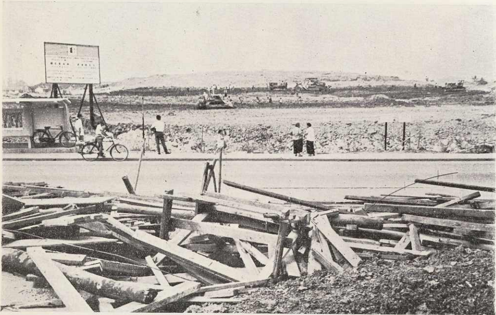
Earthmoving machines at work in Bukit Ho Swee Fire Site.
