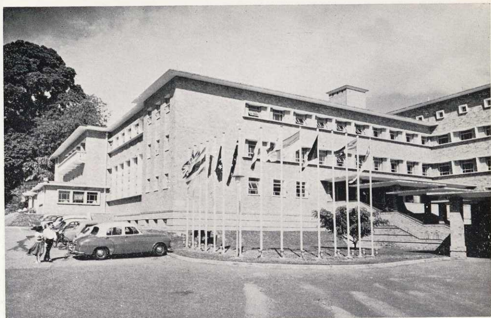
A view of the National Library where the U.N. Seminar on Urban Community Development was held in December 1962.
