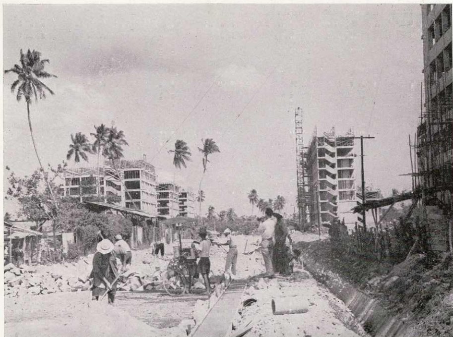
Road construction in progress for the MacPherson (S) Estate
