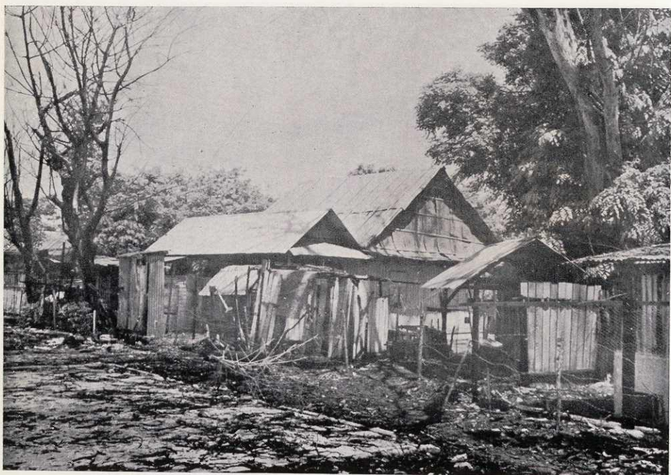
Dilapidated "Shacks" in a typical squattered area before clearance.
