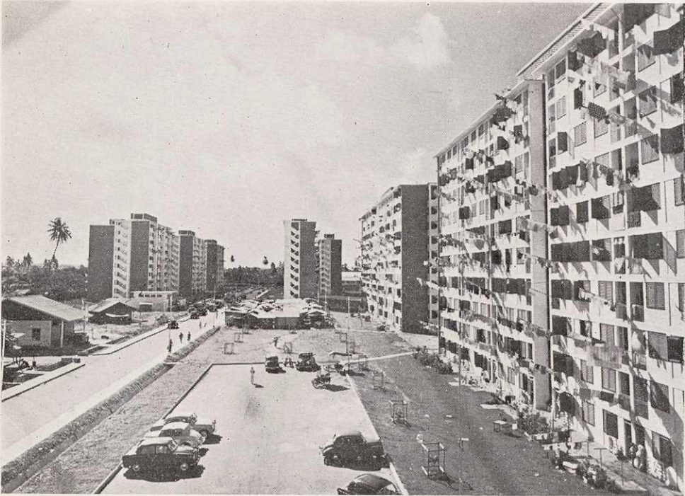
General View of the 10-storey flats from Jalan Merpati in MacPherson Road (South) Estate.
