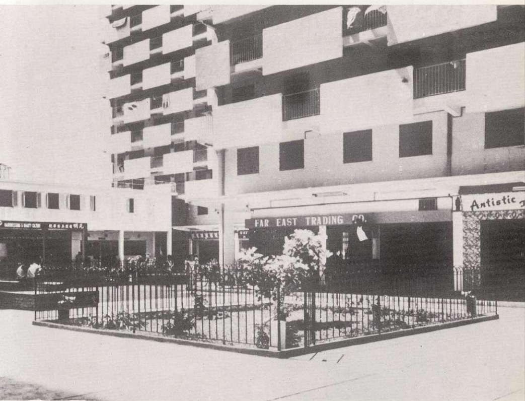
A view of the internal court of Selegie House surrounded by shopping arcades with 39 shops and a restaurant.
