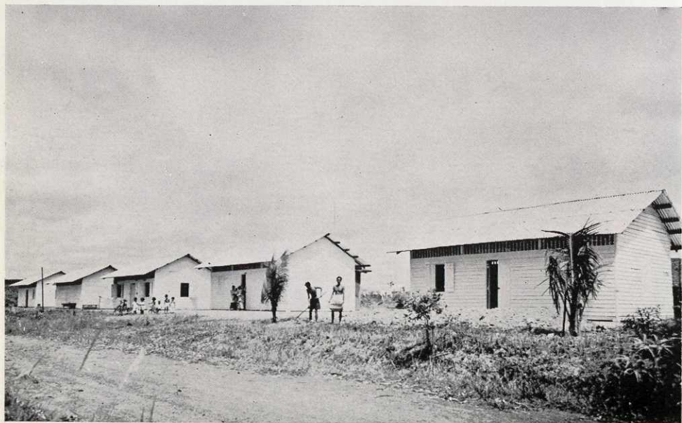
Prepared Resettlement Site with completed free basic houses to families cleared from areas required for development.
