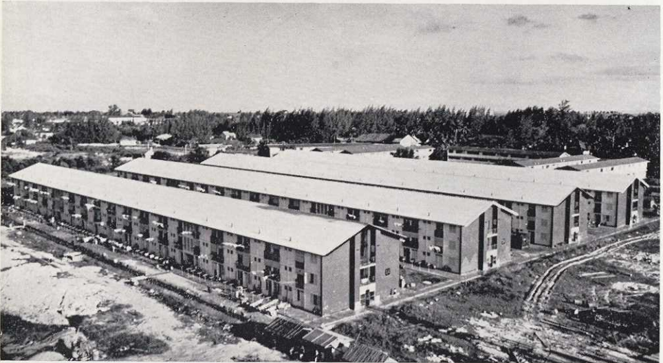
Four Blocks of 3-Storey 1-Room self-contained flats, at Kallang Estate. Rent $20/- per month.
