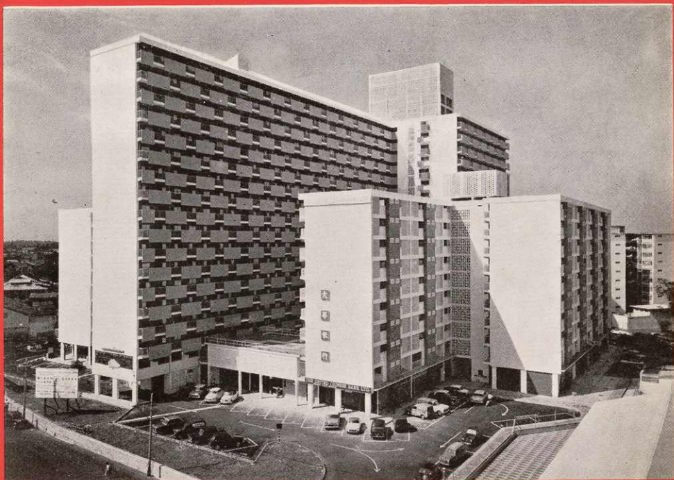
Selegie House. The first precinct of urban redevelopment in Singapore. Two blocks of 10-storey flats and a 20-storey block with 505 housing units including 39 shops and a restaurant. This 20-storey block is the tallest building constructed by the Housing Board up to date.
