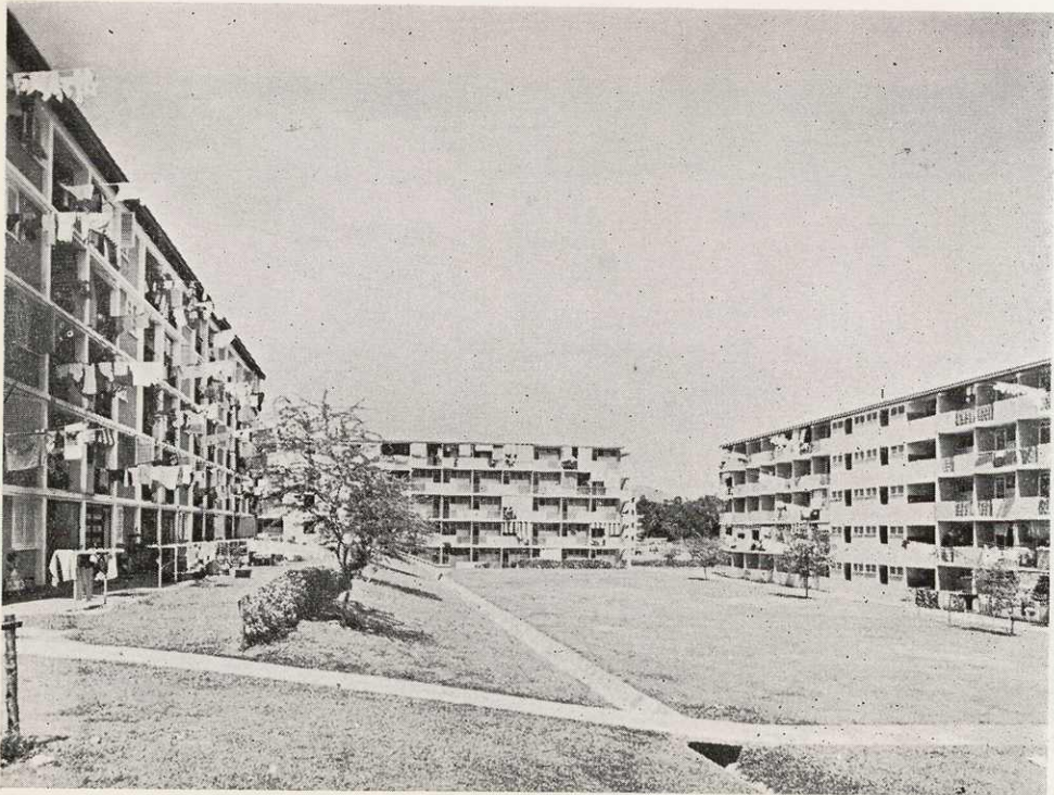
Open spaces between the buildings in Kampong Tiong Bahru Fire Site.
