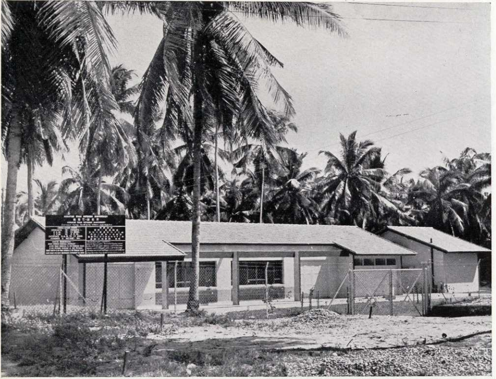
One of the Outdoor Dispensaries built by Housing & Development Board (at Somapah Road) for the Ministry of Health.
