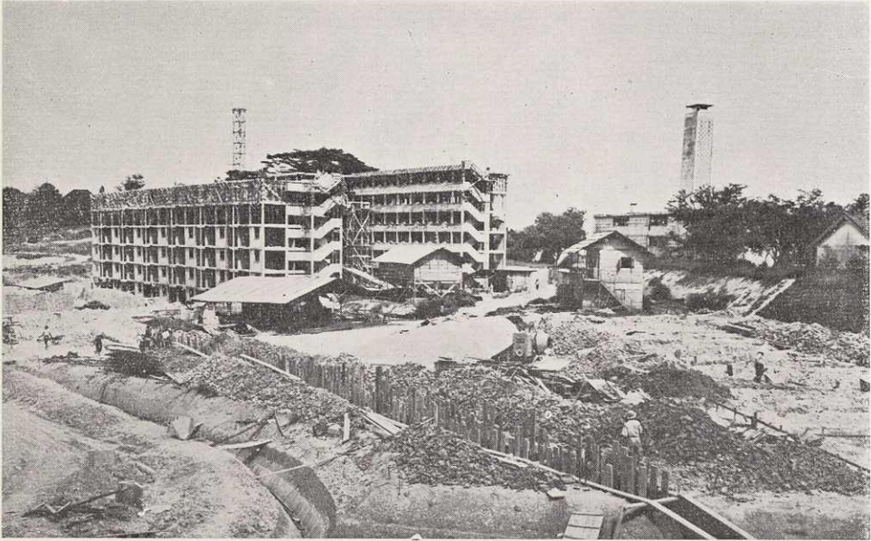
General View of Neighbourhood V, Queenstown during the early stage of construction.
