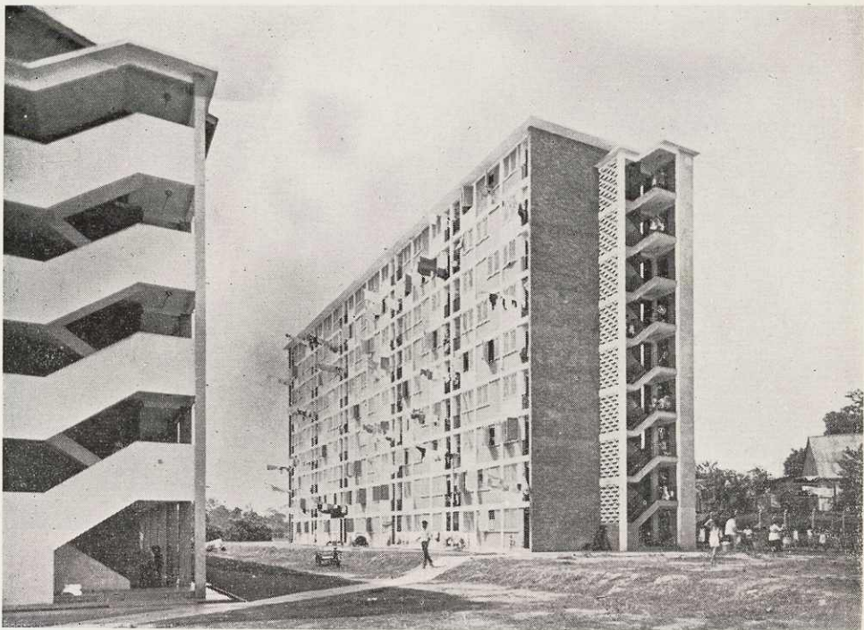
9-storey flats in Kampong Tiong Bahru Fire Site.
