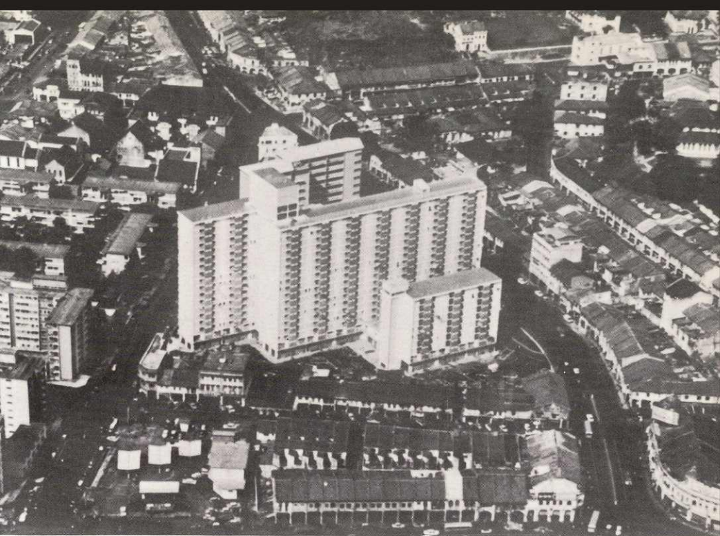
Aerial view of Selegie House.
