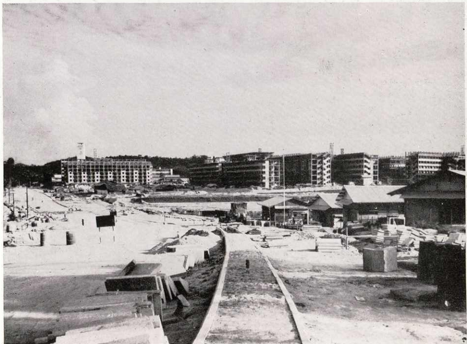
Road, roadside drains and footways being constructed at Queenstown Neighbourhood V
