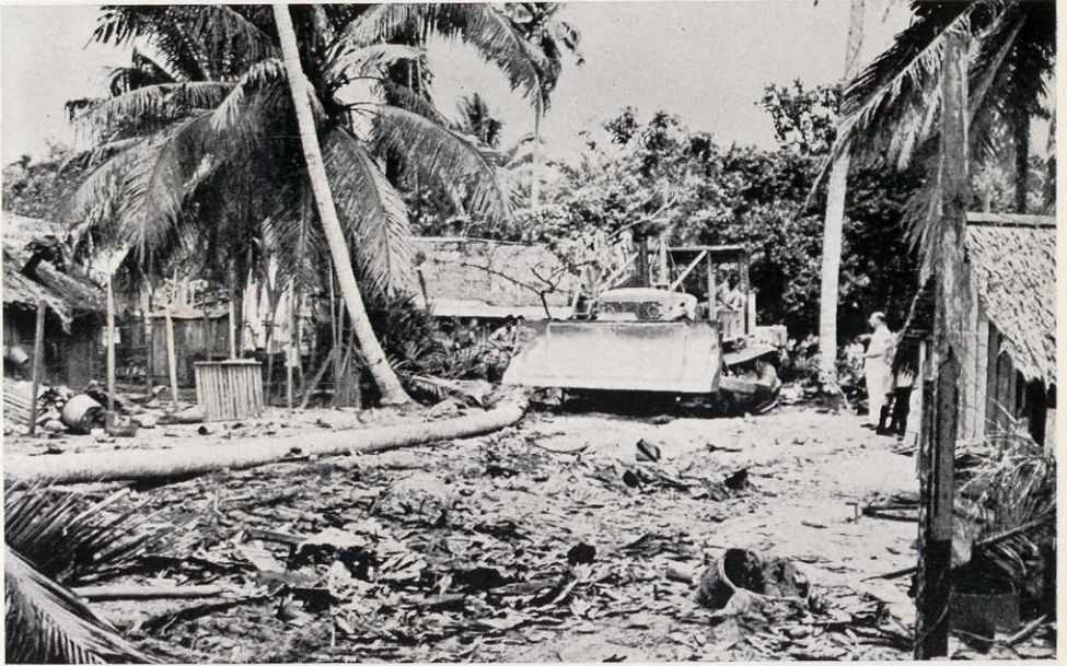
Clearance of site for Development.
