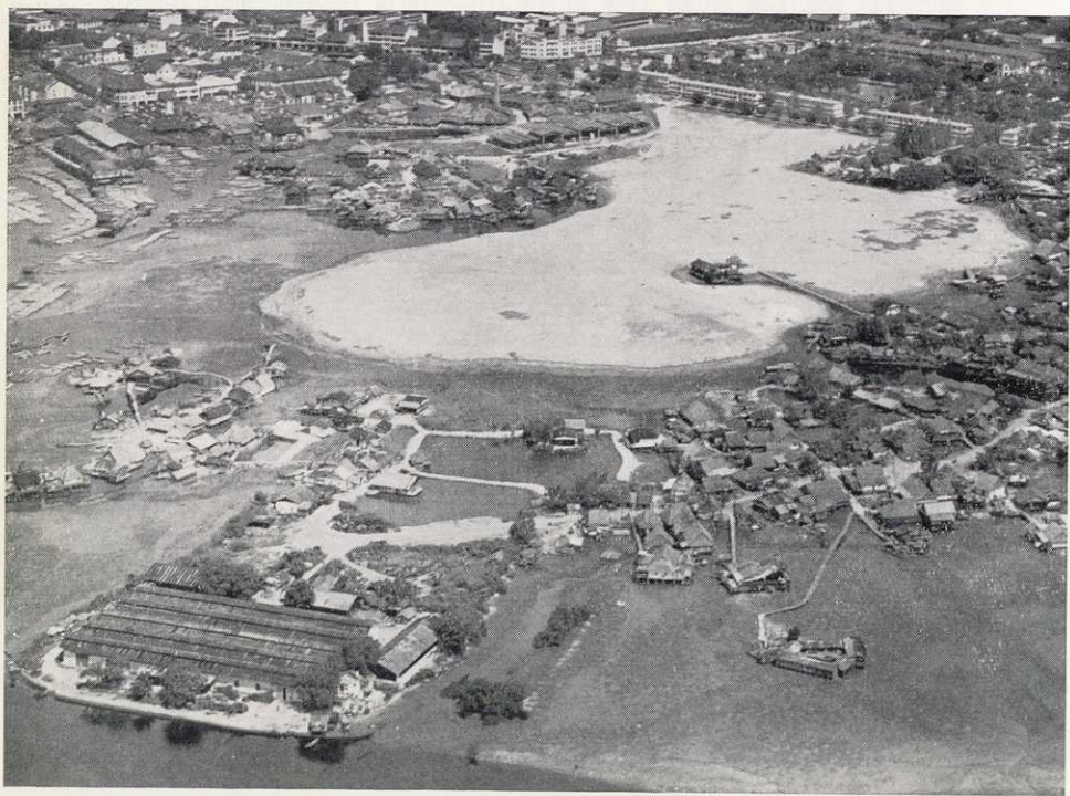
Aerial view of reclamation of Kallang Basin about 5.9 acres reclaimed when this photograph was taken.
