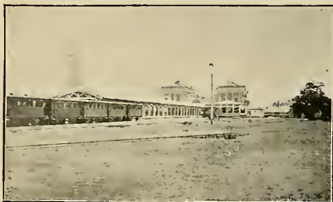
SHINBASHI STATION, TOKYO.
