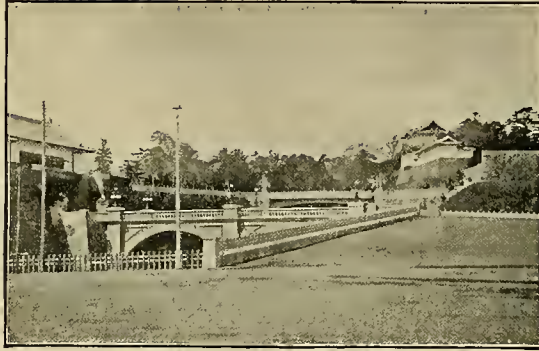
ENTRANCE TO PALACE GROUNDS.
