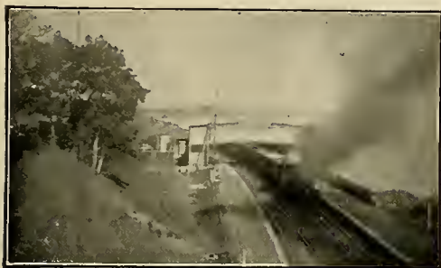
ELEVATED CROSSING FOR PASSENGERS.
