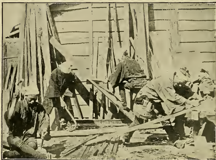
CARPENTERS AT WORK.
