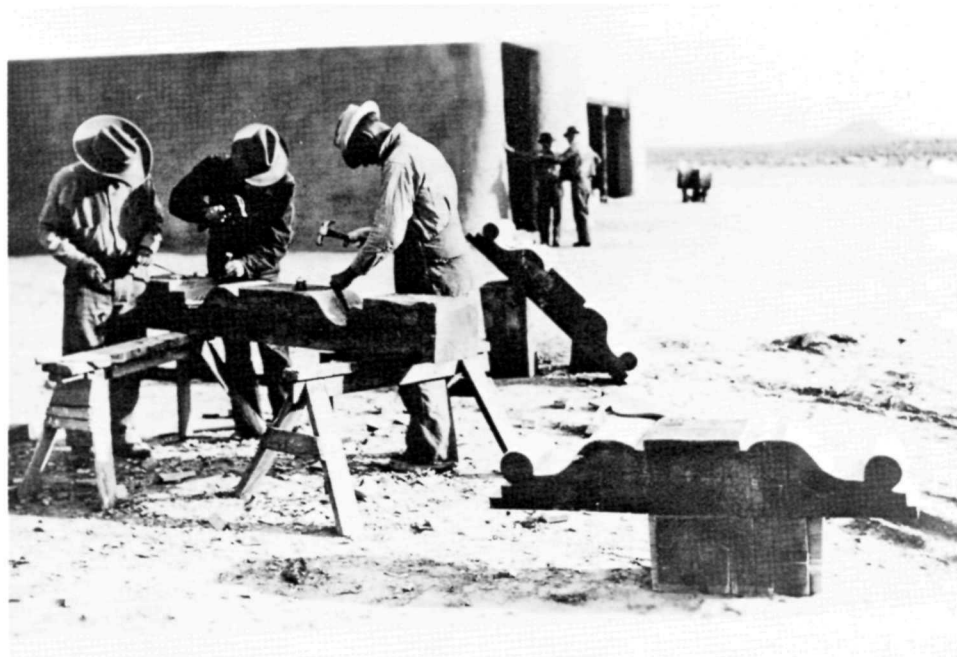
Figure 16. Hispanic woodcarvers making corbels for Visitors Center (1930s). Courtesy White Sands National Monument.
