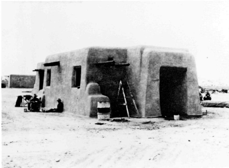
Figure 15. Adobe style of construction of New Deal Agency work crews (1930s). Courtesy White Sands National Monument.
