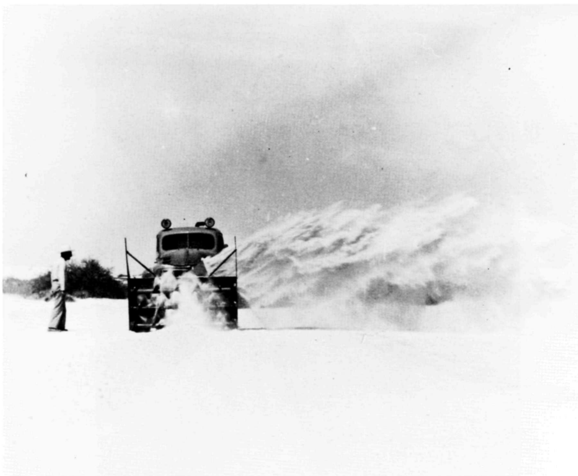
Figure 13. Blading gypsum road into the heart of the sands (1930s). Courtesy White Sands National Monument.
