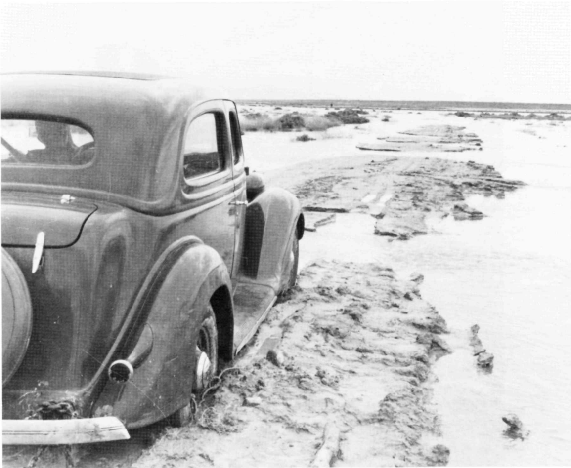
Figure 33. Clay-plated road washed out by heavy rains (1940s). Courtesy White Sands National Monument.
