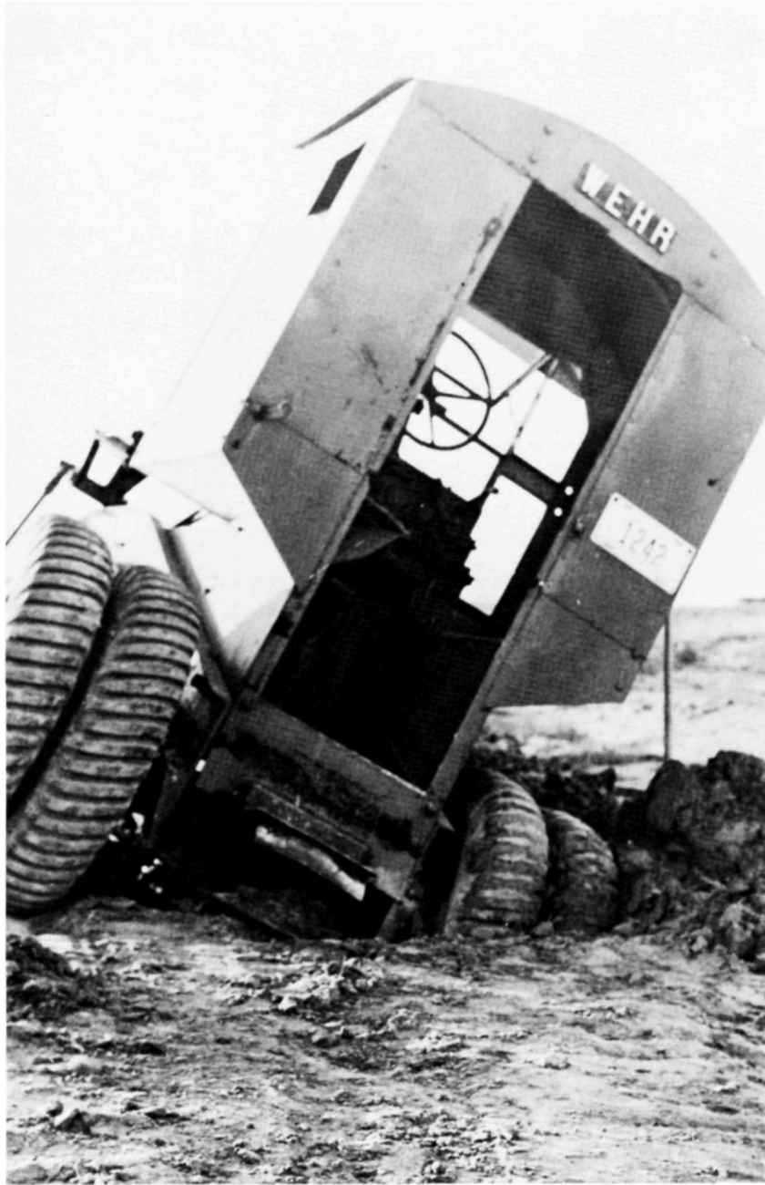
Figure 14. Hazards of road grading (1930s). Courtesy White Sands National Monument.
