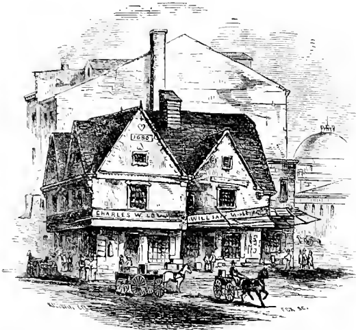
ANCIENT HOUSE IN DOCK SQUARE.
