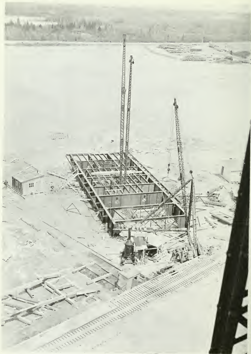
View from the water tower of Lake Shore Mines showing construction of the steel deck for the new No. 5 shaft.
