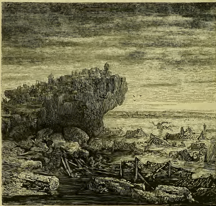
AFTER THE EARTHQUAKE.
