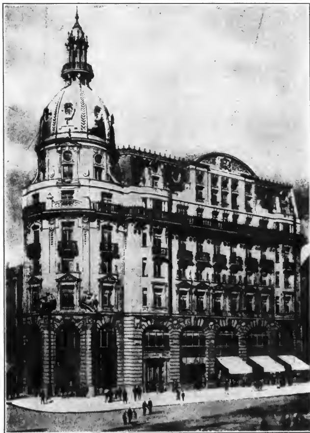
THE NEW BUILDING OF THE "JORNAL DE COMMERCIO," RIO DE JANEIRO, BRAZIL.
