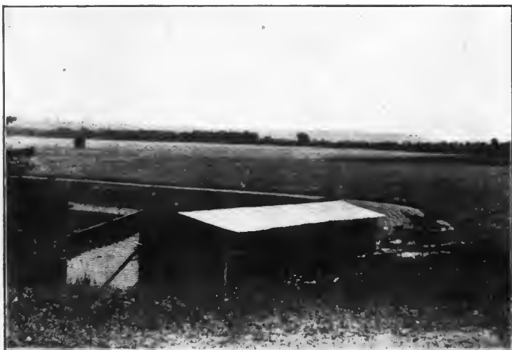
On a modern farm great benefits result from providing a suitable storage place for the ears of corn. They must be well protected from bad weather, while they have the freest ventilation to prevent the injurious effects of moisture. The picture illustrates a practical shed devised for this particular purpose. The wagon, as it comes from the field by the upper road, can be unloaded into the bin by gravity, and when it is to be loaded for transport to market the same force loads the wagon ready in the lower road.
