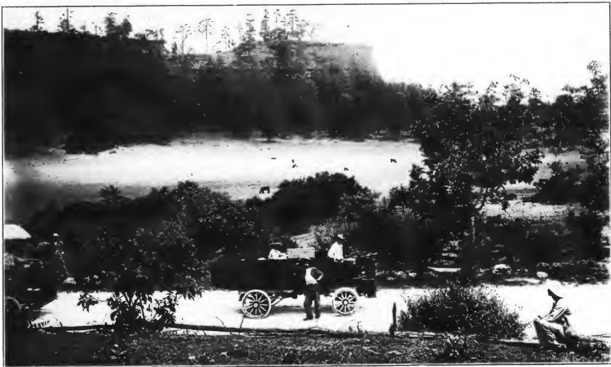
HIGHWAY FROM TEGUCIGALPA TO SAN LORENZO, HONDURAS. This road, recently completed, is one of the best highways of the Republic.
