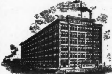
FACTORY 132 ND TO 133 RD ST & BROOK AVE
