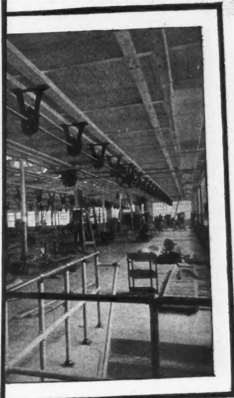
All iron work in this plant of the General Motors Corporation at Bloomfield, N. J. was first painted with two coats of Antoxide. The clean, bright airy look was then achieved by completing the finish with Du-Lite (white mill paint) which is also made by DuPont.
