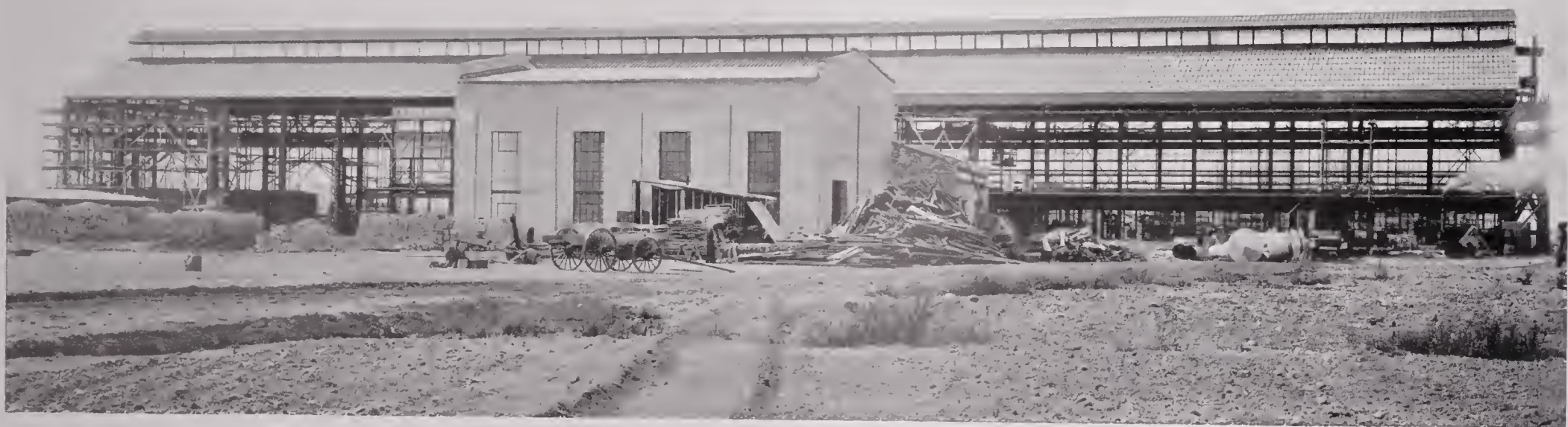
EAST SIDE OF DROP FORGE PLANT
