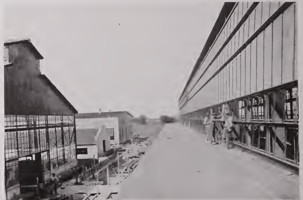
FROM HAMMER SHOP ROOF
