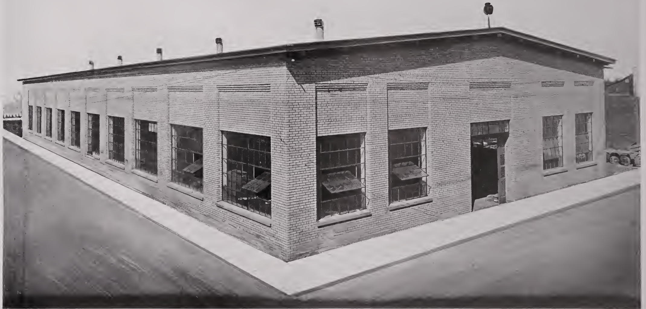
ONE OF THE UNITS OF THE DROP FORGE DEPARTMENT
