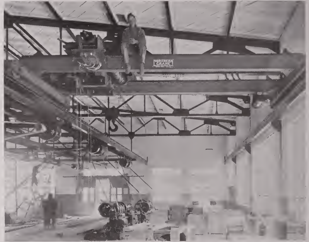
ONE OF THE THREE TON OVERHEAD CRANES
