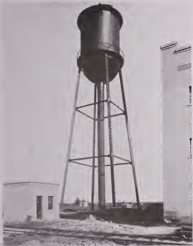
WATER TOWER AND PUMP HOUSE
