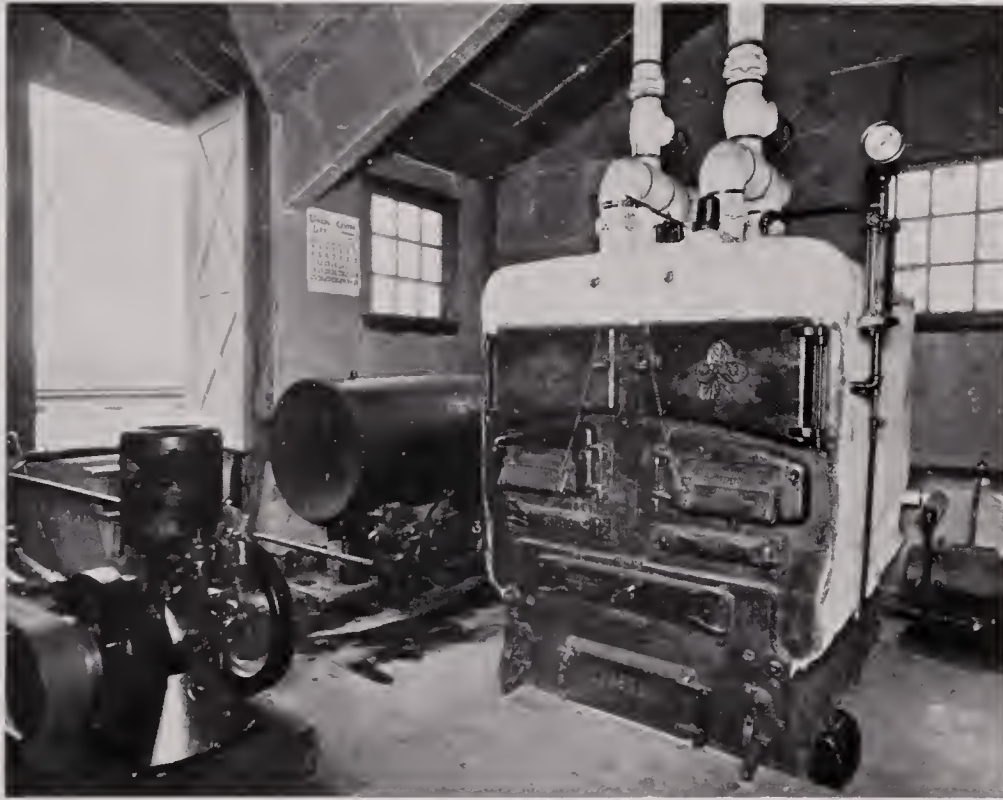
THE BOILER ROOM AND PUMP STATION
