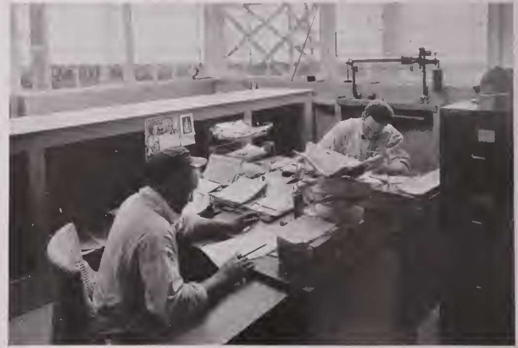
WEIGHMASTER, SHIPPING AND RECEIVING DEPARTMENT Factory Building Number Two
