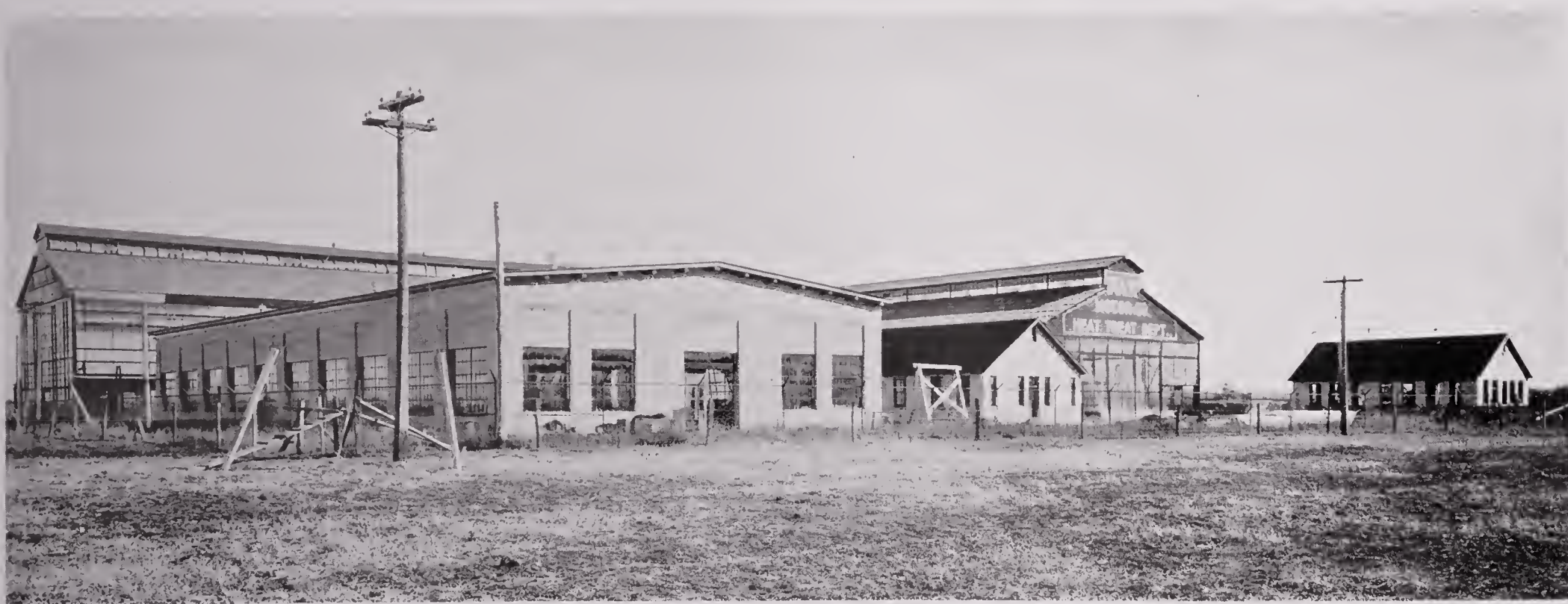
ANOTHER VIEW OF THE DROP FORGE PLANT GROUP
