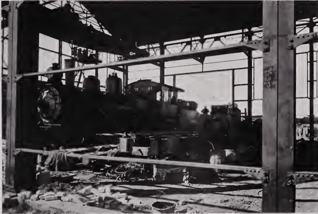
NOT A ROUNDHOUSE—JUST UNLOADING
