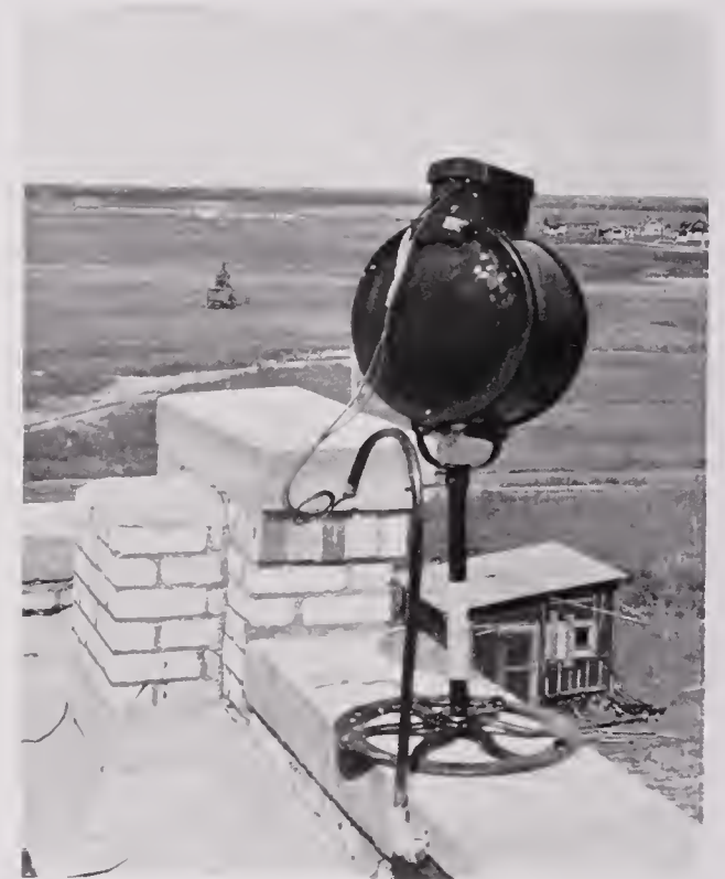
PROPERTY FLOODED BY LIGHT AT NIGHT
