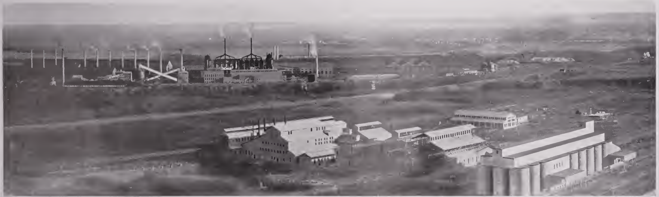
PLANT OF THE MINNESOTA STEEL COMPANY, AT DULUTH. (SEE CHART B.)
