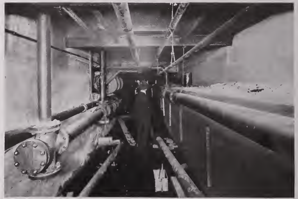
THESE LONG TUNNELS RUN FROM THE POWER HOUSE TO ALL BUILDINGS
