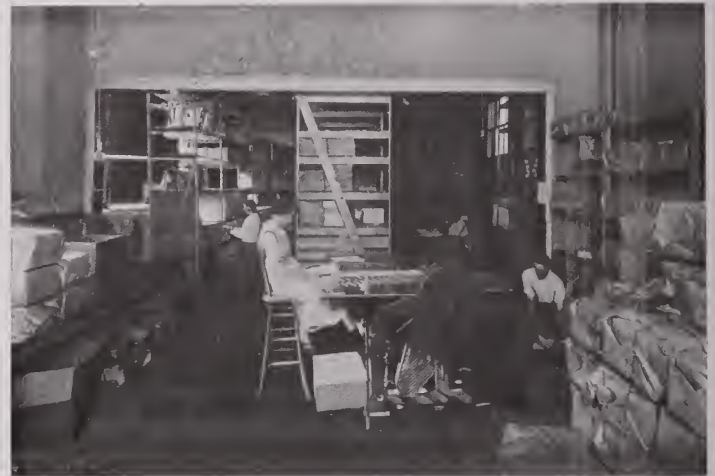
STATIONERY AND PRINTING STOCK ROOM Board of Education Building
