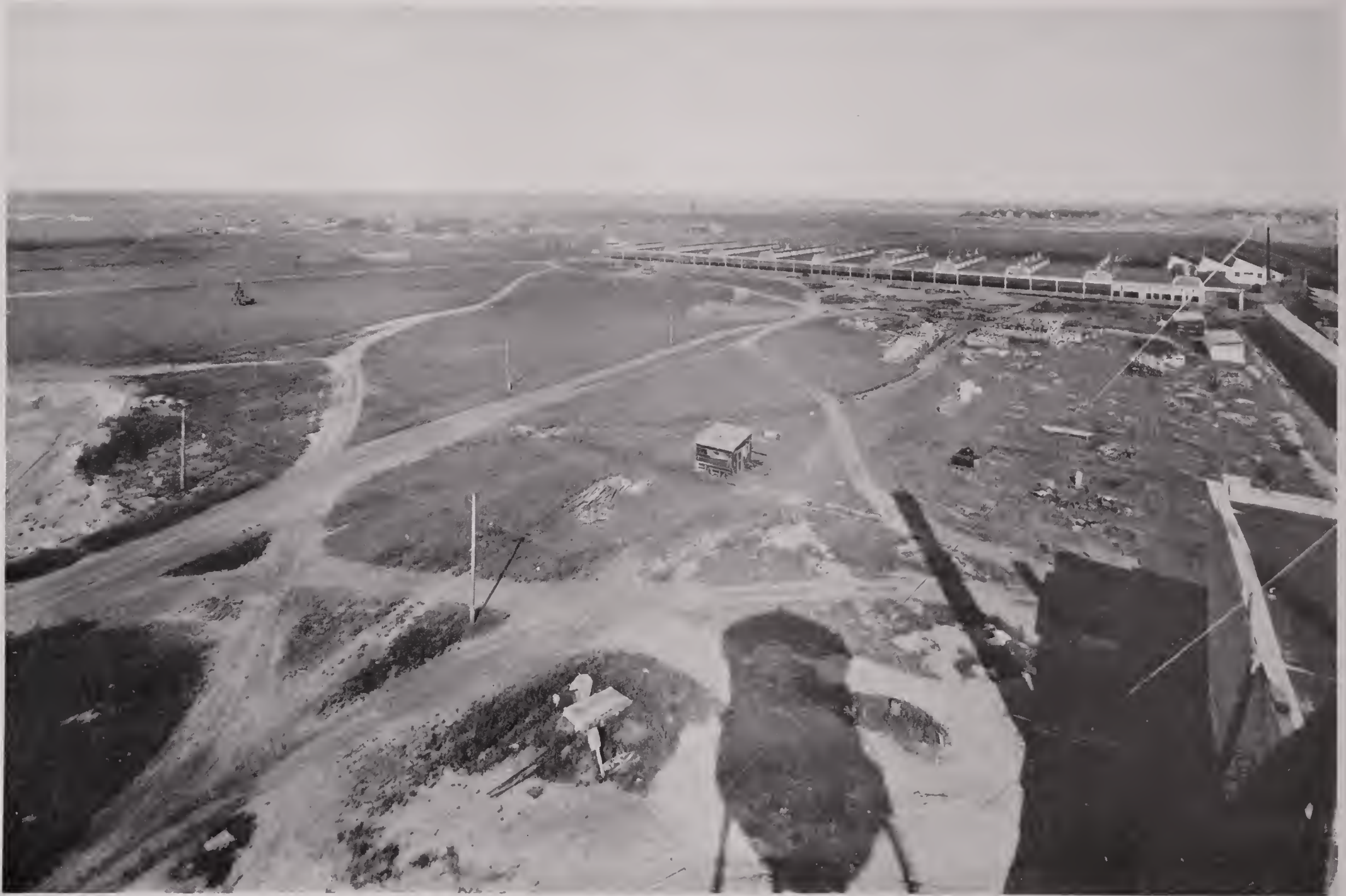
VIEW FROM THE WATER TOWER
