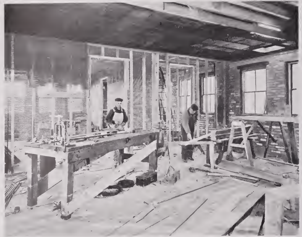
INTERIOR LABORATORY BUILDING DURING CONSTRUCTION
