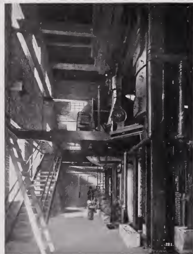
ALONG SOUTH SIDE BOILER ROOM
