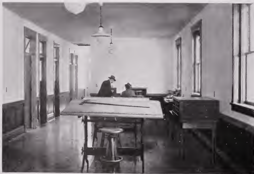
DRAFTING ROOM DROP FORGE DEPARTMENT Drop Forge Office Building
