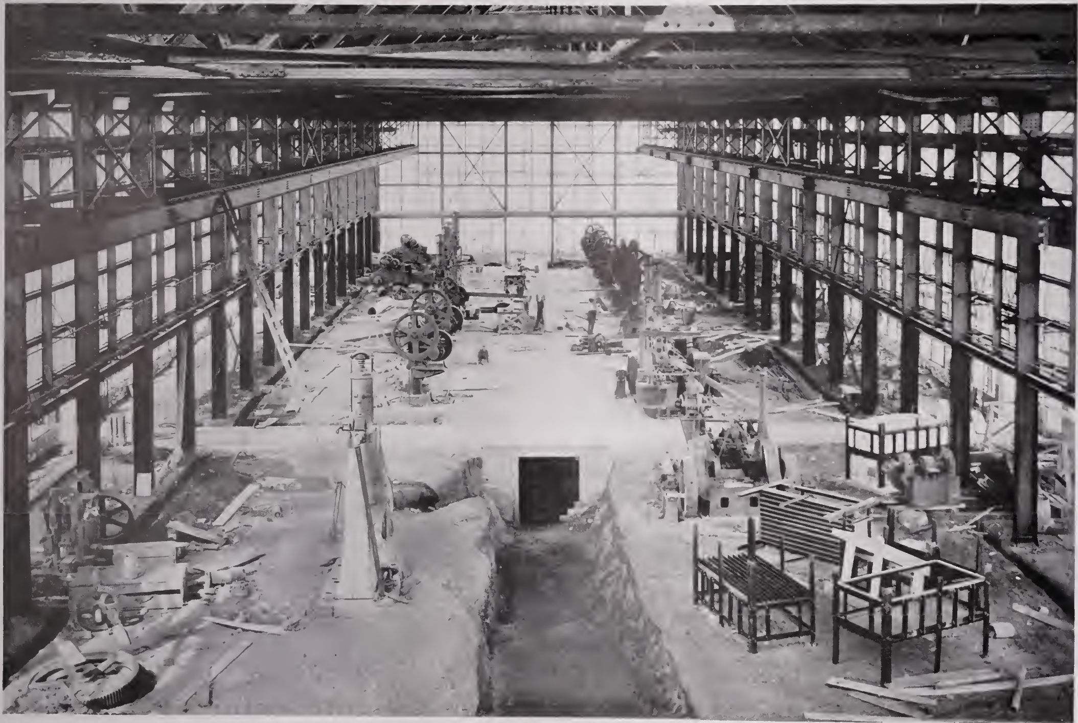
LOOKING NORTH IN HAMMER SHOP
