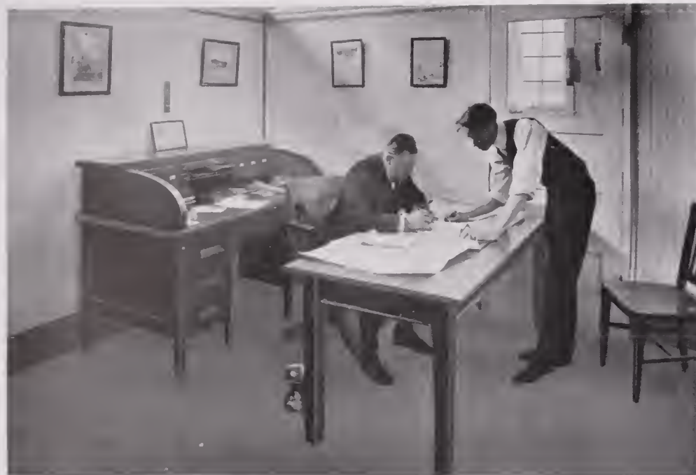
TRACTOR DESIGNING ENGINEER'S OFFICE Experimental Engineering Building
