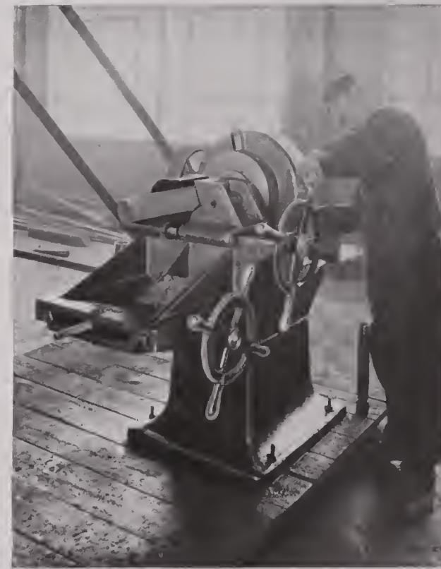
OSTER PIPE THREADING MACHINE
