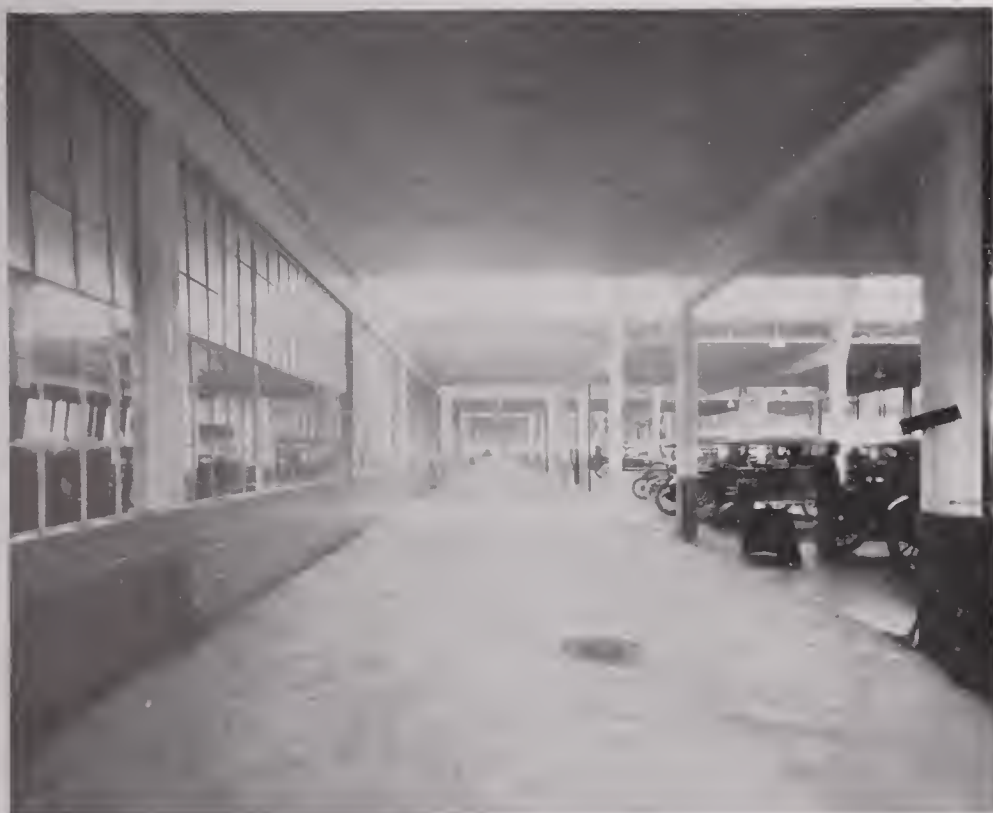
LOOKING DOWN THE MAIN AISLE
