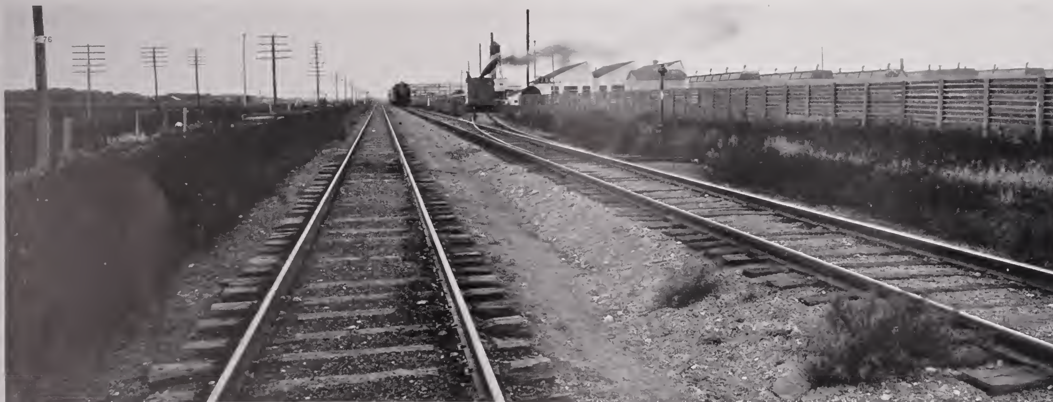
THE RAILROAD ENTRANCE TO THE PLANT
