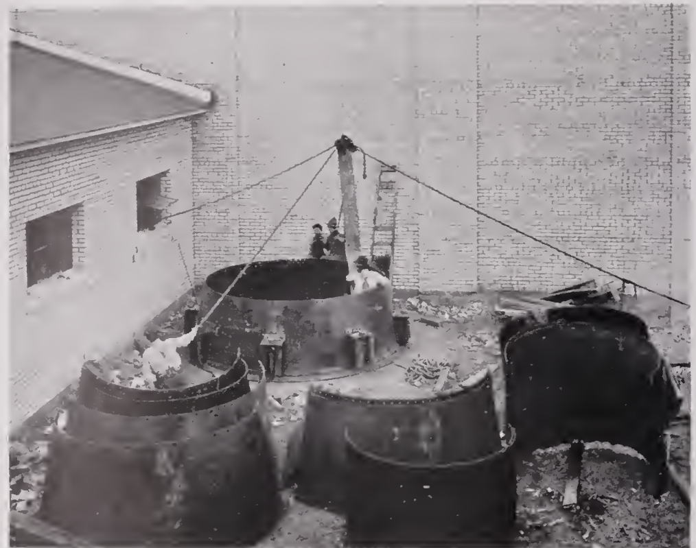
ERECTING FORGE POWER PLANT STACK
