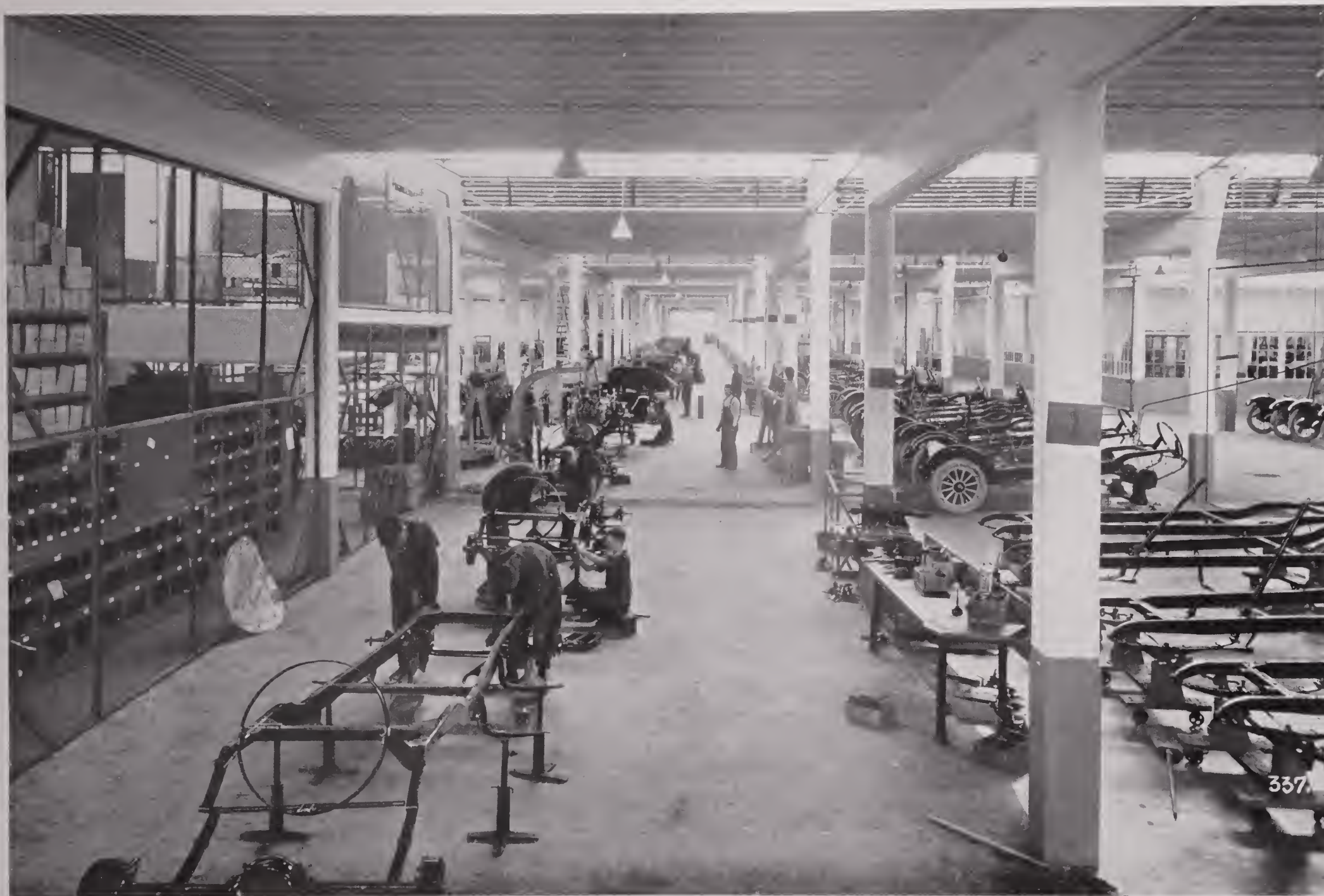
LOOKING DOWN THE MAIN ASSEMBLY LINE IN FACTORY BUILDING NUMBER TWO
