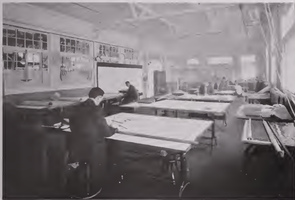
DRAFTING ROOM—ENGINEERING DEPARTMENT Experimental Engineering Building
