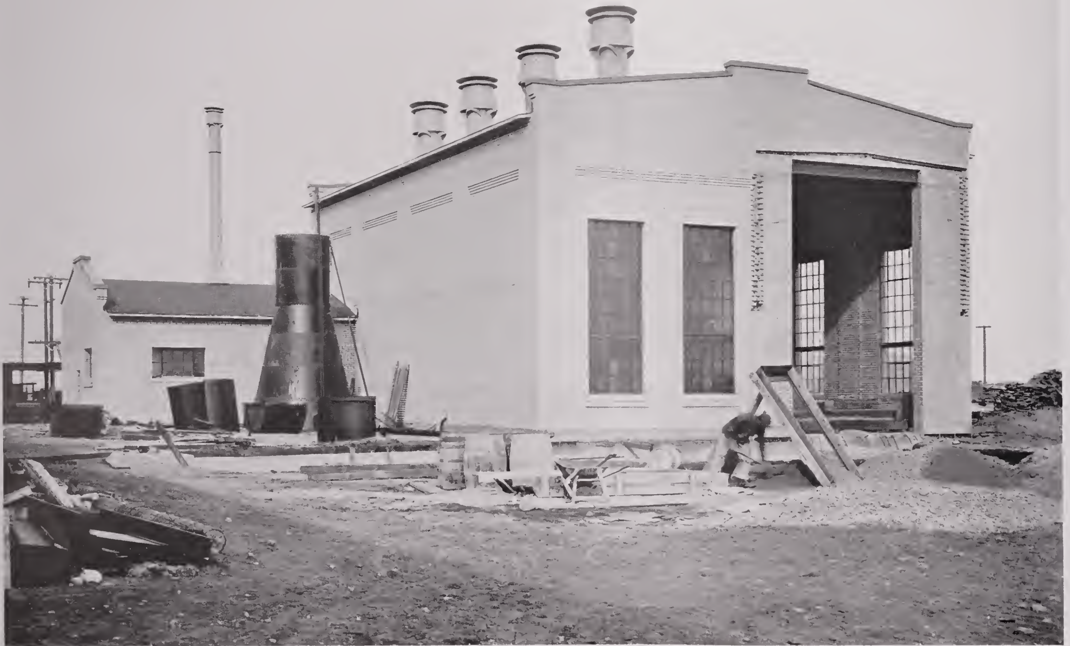
STEAM BOILER PLANT OF DROP FORGE DEPARTMENT
