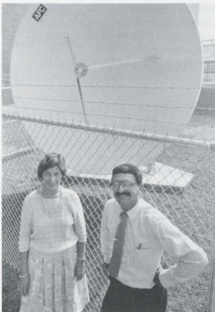
SATELLITE DISH... A new satellite dish for receiving special teleconferencing programming was recently installed behind the College of Science by Instructional Media Services (IMS). The dish will be used mainly for instructional purposes and will make RIT the only college in the Rochester area to have teleconferencing capabilities. On left is IMS Director Joan Green, and Robert Gascon, IMS engineering manager who oversaw the installation of the system.
