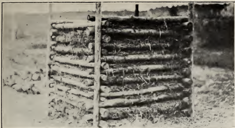
FIG. 1.—CONSTRUCTION OF CRIB.
