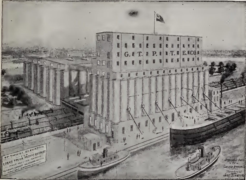
Grand Trunk Pacific Railway Co. Elevators at Fort William, Ont. Capacity 3,500,000 Bushels.
