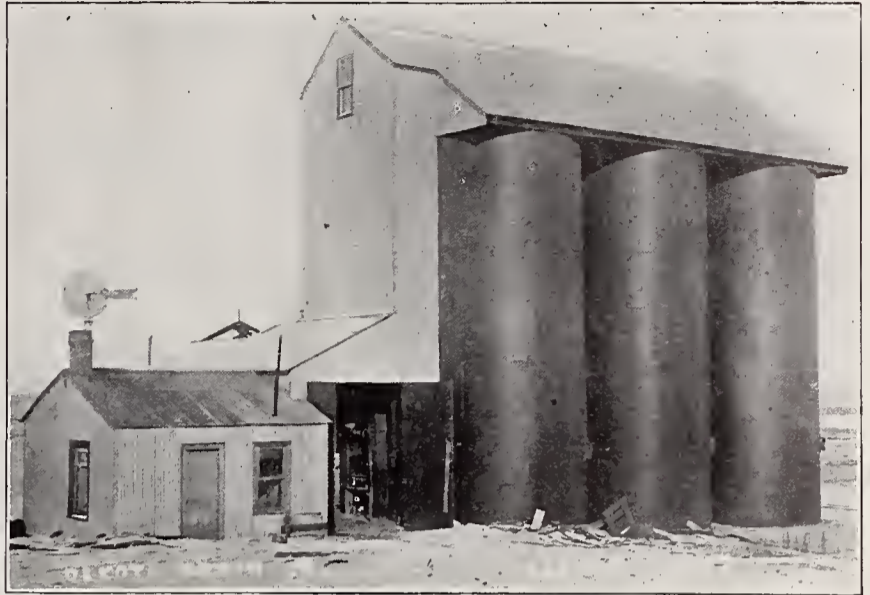
30,000 Bushel Steel Elevator Built for Dakota Grain Co. at Alfred, N. D.
